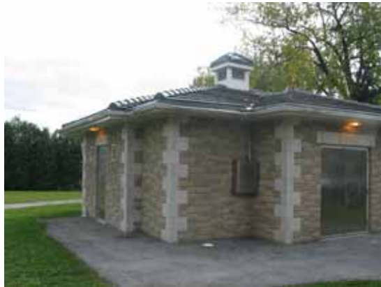
1. Wetwell / drywell station
