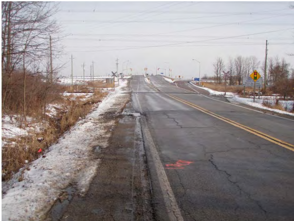
Photo 6: CP Railway, looking East. [Borehole 12-21]
