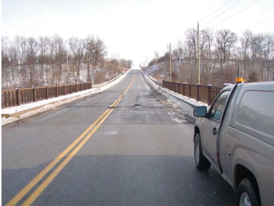
Photo 3: Sixteen Mile Creek (West Branch), looking East. [Borehole 12-07 and 12-08]
