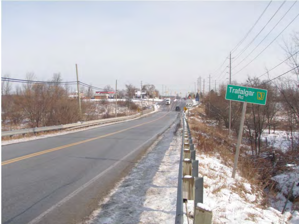
Photo 5: Sixteen Mile Creek (East Branch), looking East. [Borehole 12-17 and 12-18]
