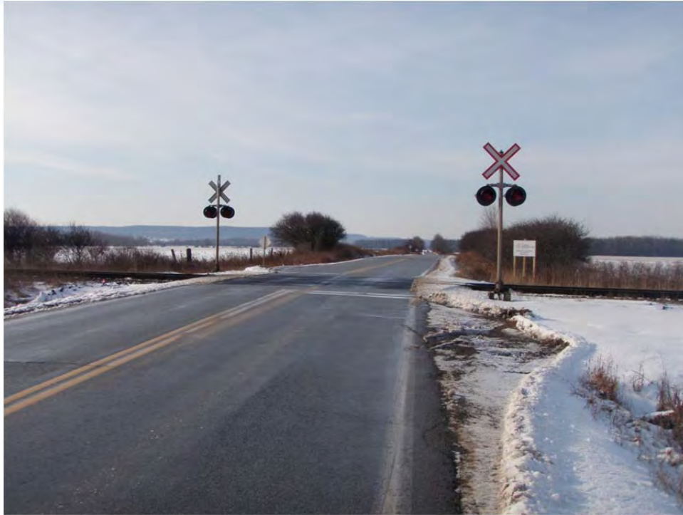
Photo 1: CN Railway, looking East [Borehole 12-02 and 12-03, to be drilled]
