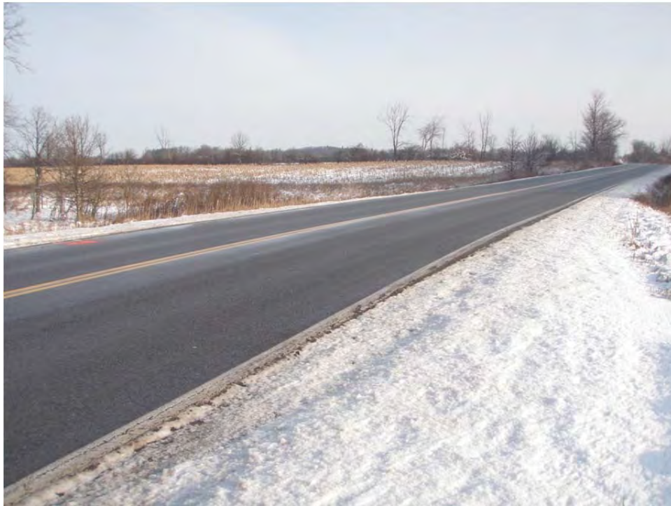
Photo 2: West tributary of Sixteen Mile Creek, looking East [Borehole 12-05]
