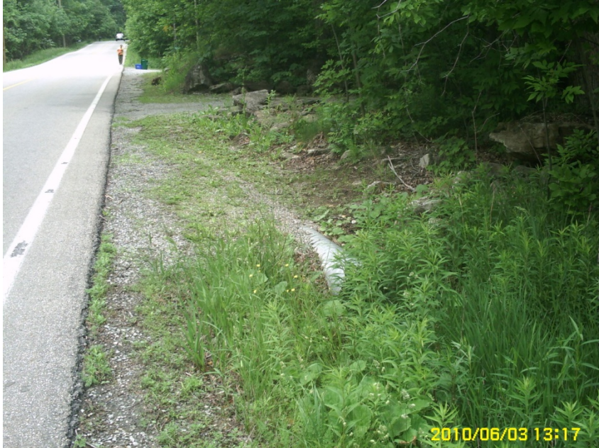
7. Drainage feature with culverts along northeast side of road.
