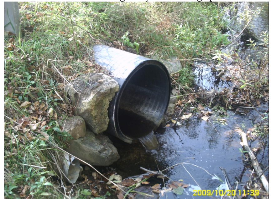
4. Existing culvert under Derry Road
