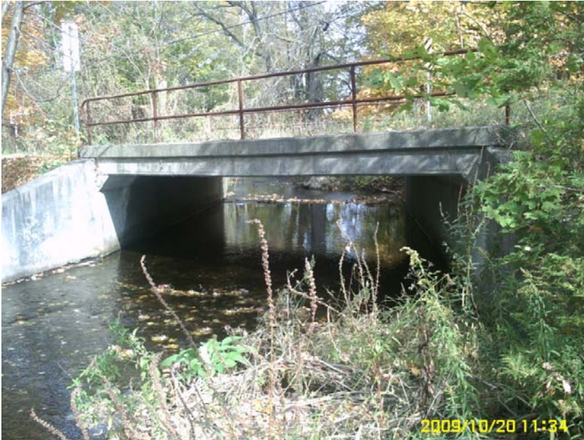
1. Kilbride Creek at McNiven Road culvert facing downstream
