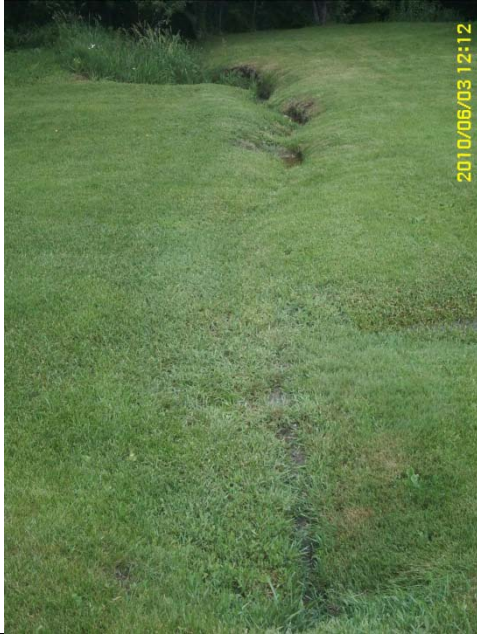
21. Small channel in-between residential properties, mowed and not stable at bend
