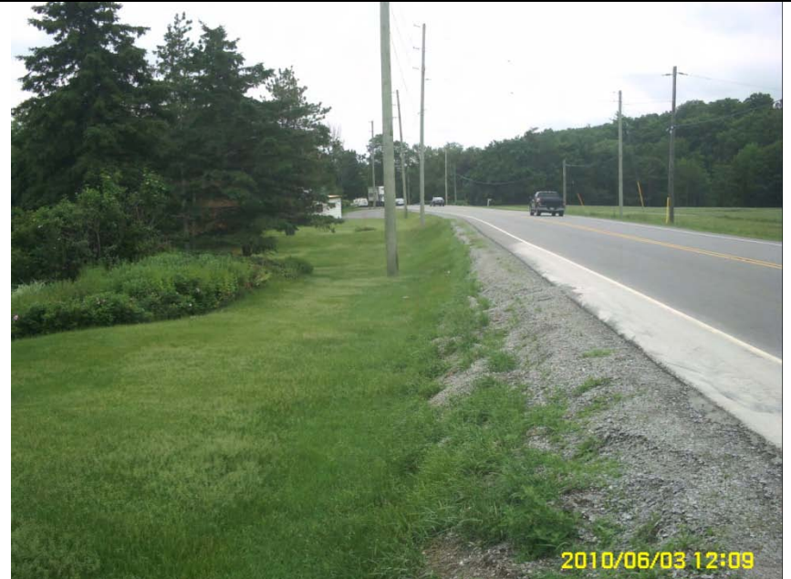
20. East side, further down the proposed road improvement, gravel slumping
