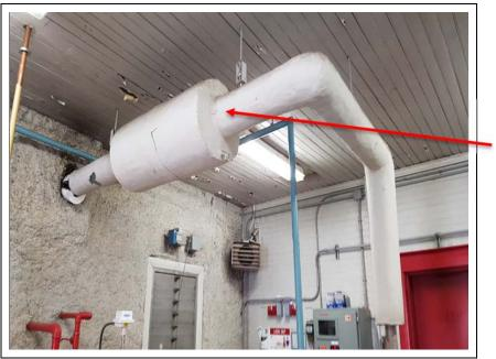
P2 – Junction Street Pumping Station View of non-asbestos containing parging cement on mechanical pipe that was observed and sampled.
