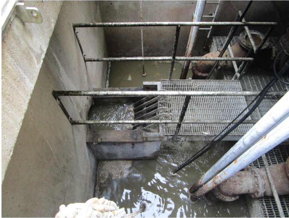
Figure 3-2: Bar screen with a buildup of material
