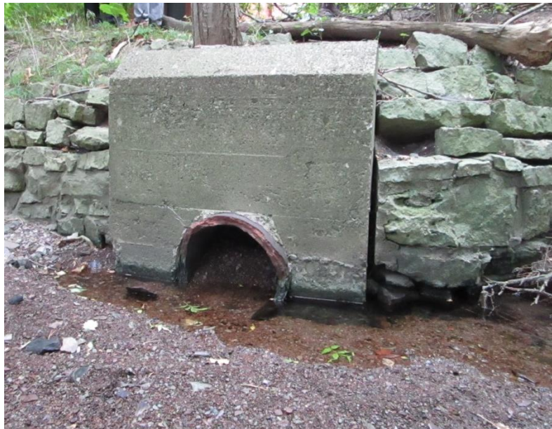
Figure 3-5: Junction Street WWPS overflow pipe discharge pipe at Rambo Creek
