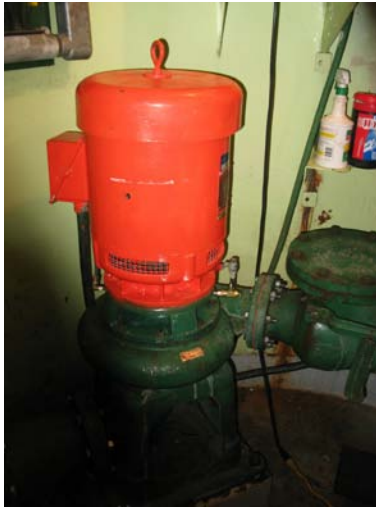
Photo 14 Vertical – Centrifugal Pump
