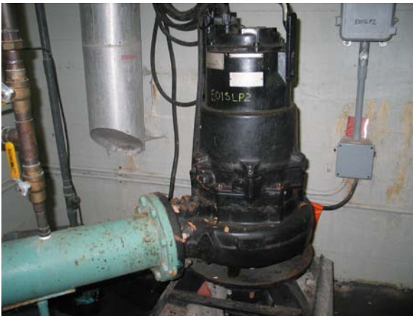
Photo 21 Submersible Pump
