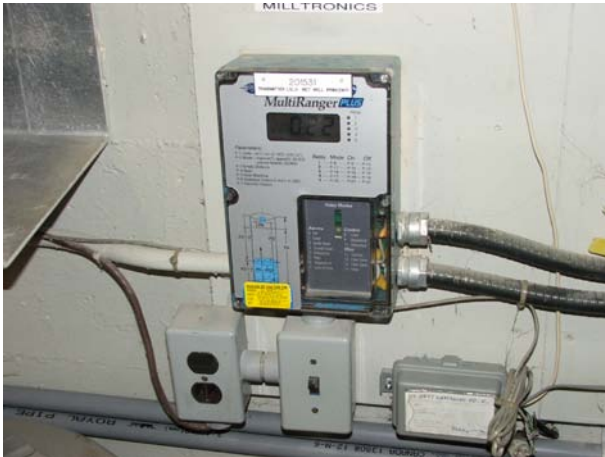
Photo 25 Level Transmitter
