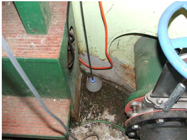
Photo 25 Process Instrumentation – Overflow Float
