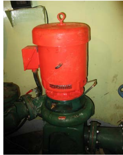
Photo 15 Vertical – Centrifugal Pump
