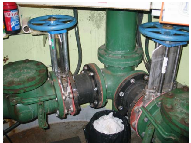
Photo 12 Discharge Header
