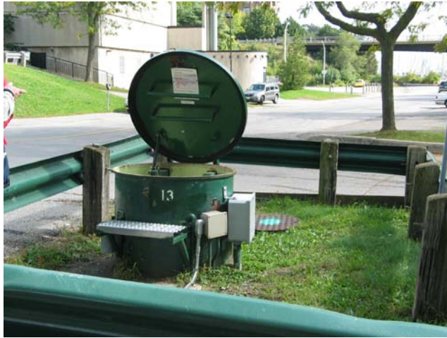
Photo 1 Prefabricated Chamber with Adjacent Wet Well
