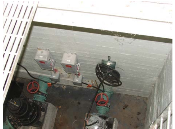
Photo 20 Two (2) Submersible Pumps in the Dry Well
