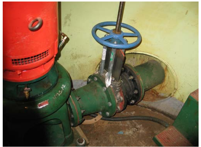
Photo 8 Pump and Suction Piping
