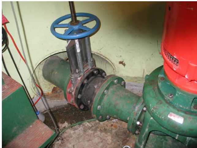
Photo 9 Pump and Suction Piping
