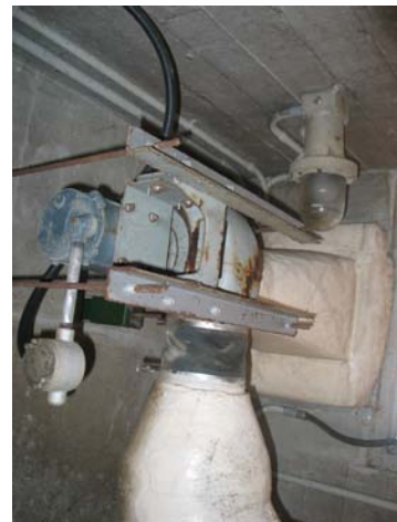
Photo 18 Wet - Well Mechanical Ventilation
