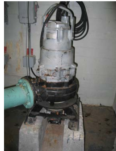
Photo 22 Submersible Pump
