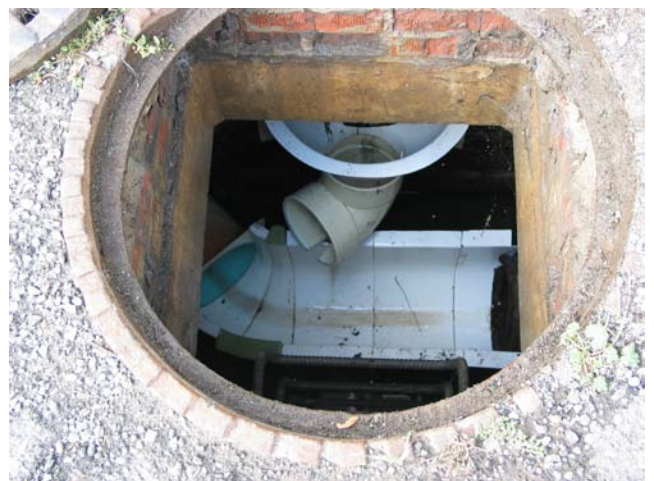
Photo 6 Overflow Chamber
