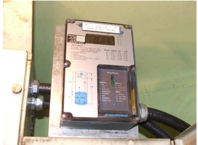
Photo 24 Process Instrumentation - Level Transmitter
