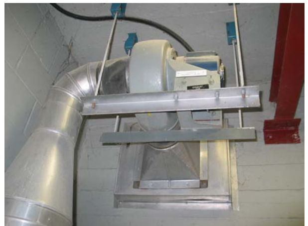
Photo 12 Dry Well Pump Floor Area - Air Supply Fan
