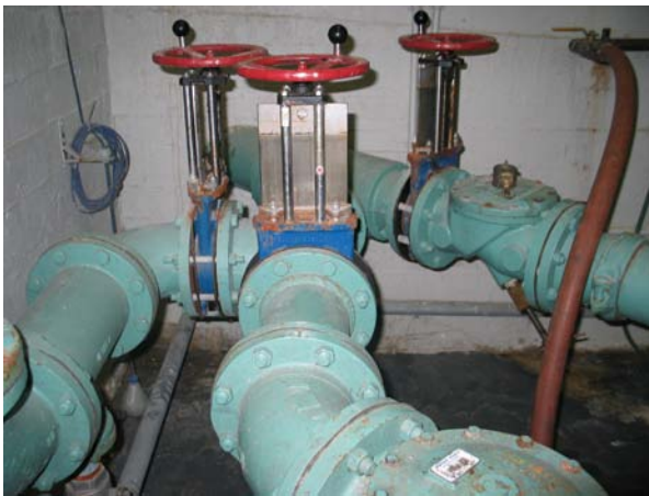
Photo 17 Pump and Suction Piping
