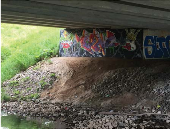
Photo 13: slumping rip-rap under Derry Road bridge.
