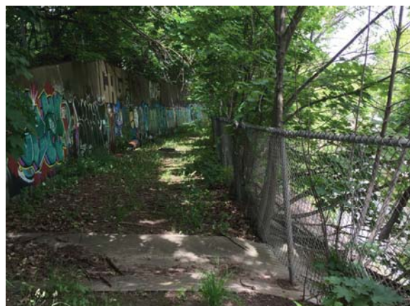
Photo 23: Stormwater passage and retaining wall adjacent to hardened creek channel in area of potential creek crossing.
