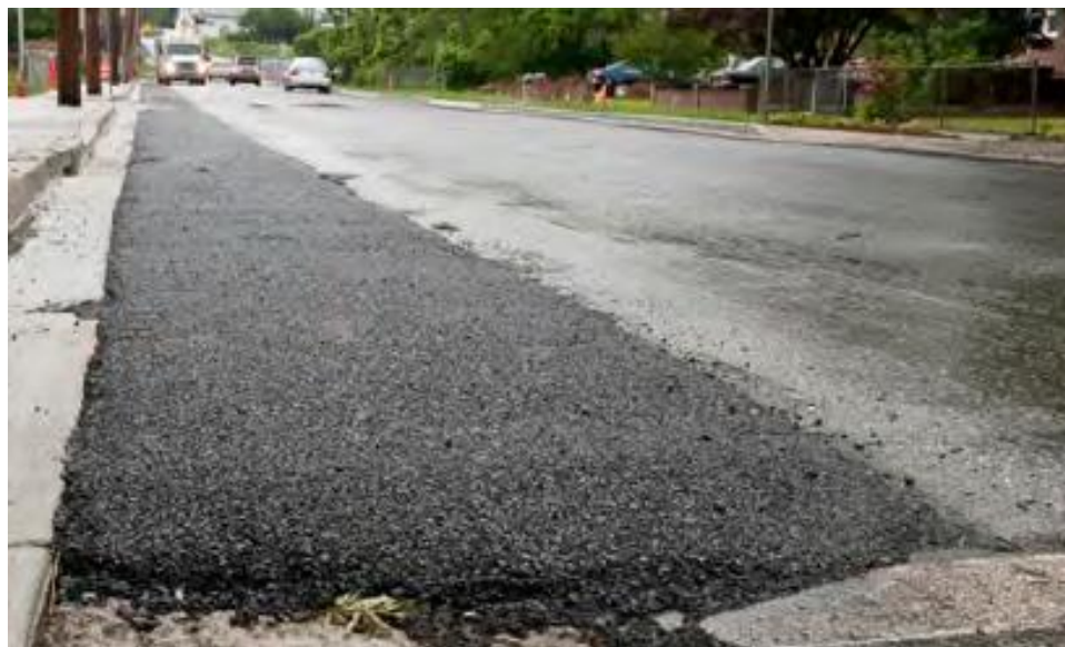
Figure 6-12 – Example of Porous Asphalt Bicycle Lane (From Credit Valley Conservation, Grey to Green Road Retrofits, 2014)
