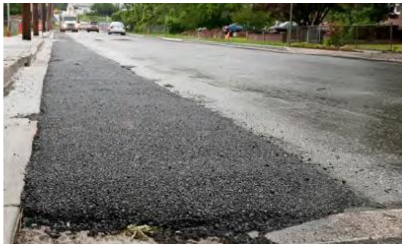
Figure 5-3 – Example of Porous Asphalt Bicycle Lane (from Credit Valley Conservation, Grey to Green Road Retrofits, 2014)
