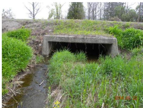
Figure 2-1 – Main Crossing Culvert
