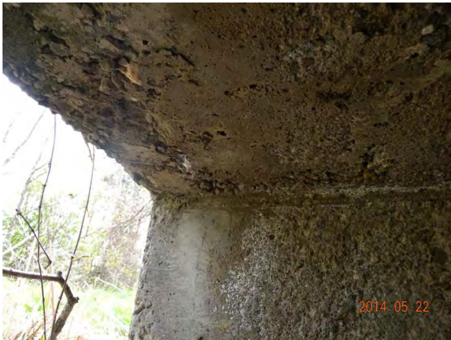
Photograph No. 4: 8662: Deck soffit at Southeast corner of structure
