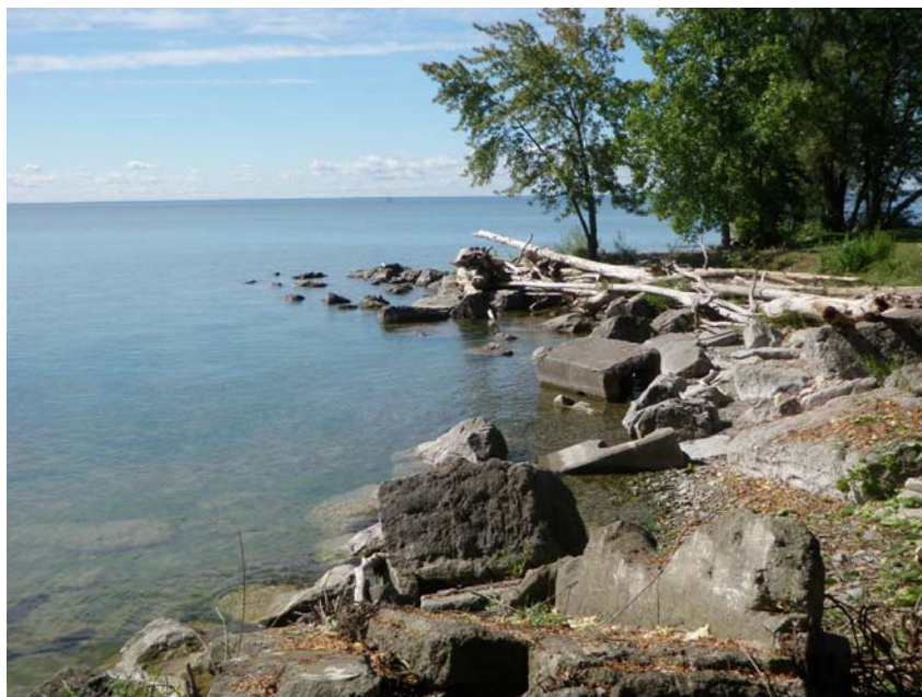
Image 9: Existing shoreline conditions from Oakville Water Treatment facility with evidence of displaced concrete block along waterline, looking west.
