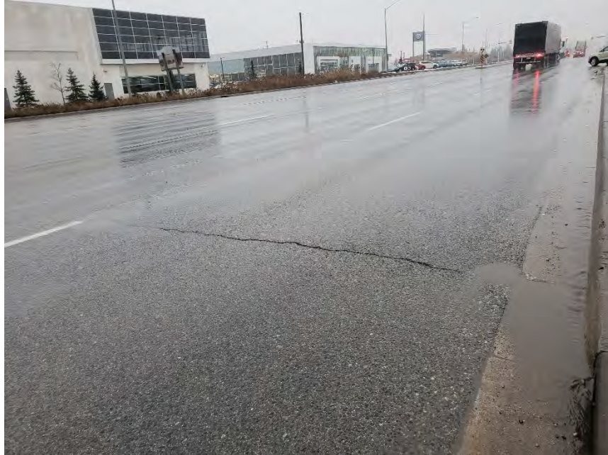
Photograph 9 – Region Road 25, Northbound, 70m north of High Point Drive, looking north, showing slight to moderate transverse cracking.
