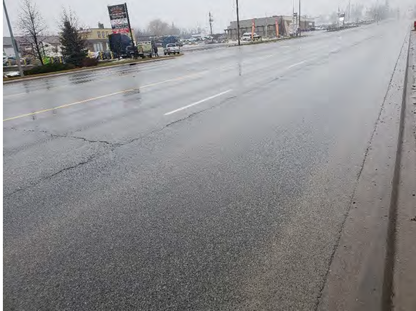
Photograph 23 – Region Road 25, Northbound, 110m north of Peddie Road, looking north, showing slight to moderate longitudinal and transverse cracking.
