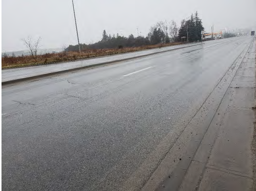
Photograph 13 – Region Road 25, Northbound, 70m north of James Snow Parkway, looking north, showing slight transverse cracking and slight ravelling.
