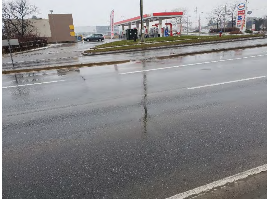
Photograph 5 – Region Road 25, Northbound, 20m South of Chisholm Drive, looking north, showing slight transvers cracking and slight wheel track rutting.
