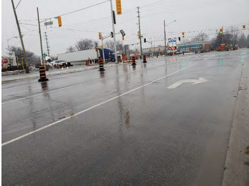
Photograph 1 – Region Road 25, Southbound, 10m North of Steeles Avenue East, looking south, showing few moderate wheel track cracking and transverse cracking.
