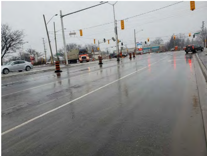
Photograph 2 – Region Road 25, Southbound, 20m North of Steeles Ave, looking south, showing slight to moderate longitudinal cracking and slight ravelling.
