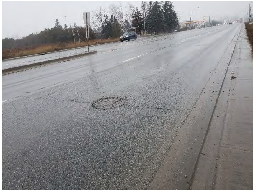
Photograph 14 – Region Road 25, Northbound, 100m north of James Snow Parkway, looking north, showing slight transverse cracking around the maintenance hole.
