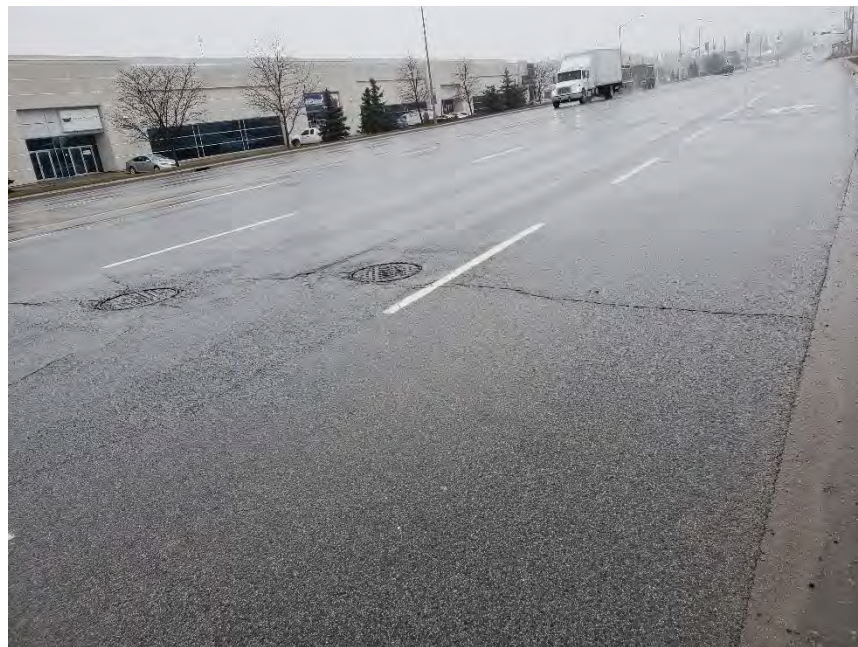
Photograph 18 – Region Road 25, Northbound, 200m south of Peddie Road, looking north, showing slight to moderate transverse and random cracking around the maintenance holes and slight ravelling.
