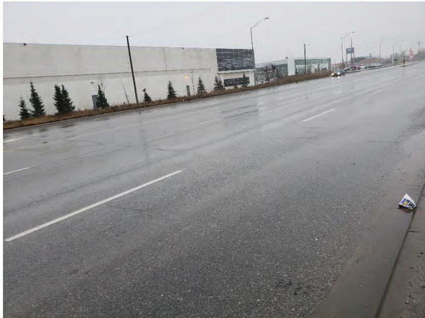
Photograph 8 – Region Road 25, Northbound, 30m north of High Point Drive, looking north, showing slight longitudinal and transverse cracking.
