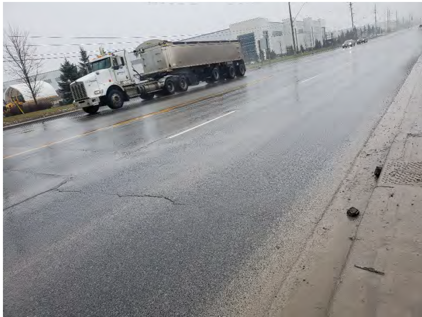
Photograph 24 – Region Road 25, Southbound, 110m south of 5 Sideroad, looking south, showing slight to moderate longitudinal and transverse cracking.
