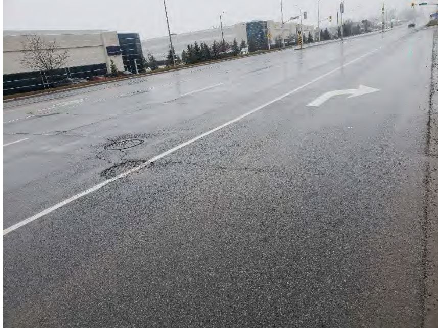
Photograph 19 – Region Road 25, Northbound, 70m south of Peddie Road, looking north, showing slight to moderate transverse and random cracking around the maintenance holes.
