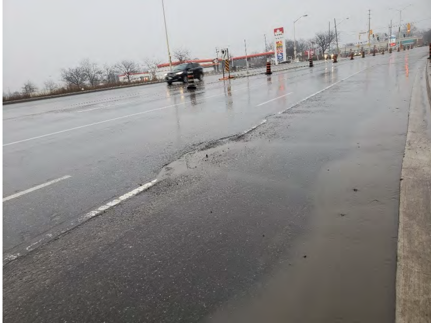
Photograph 3 – Region Road 25, Southbound, 100m North of Steeles Ave, looking south, showing slight pothole and slight to moderate ravelling.
