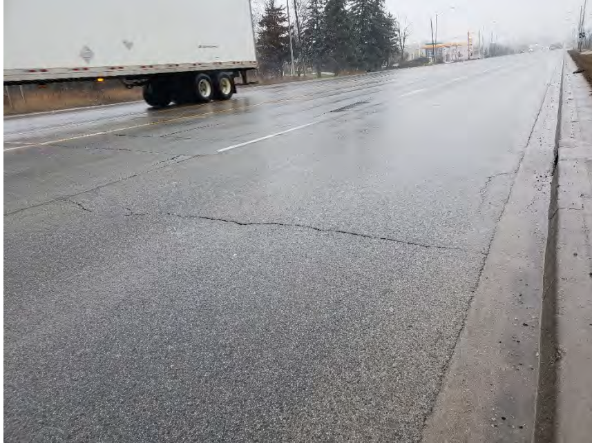
Photograph 15 – Region Road 25, Northbound, 110m north of James Snow Parkway, looking north, showing slight to moderate longitudinal and transverse cracking.
