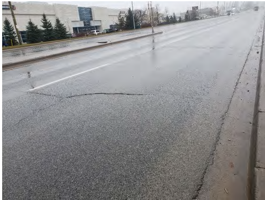
Photograph 20 – Region Road 25, Northbound, 15m north of Peddie Road, looking north, showing slight to moderate longitudinal and transverse cracking.
