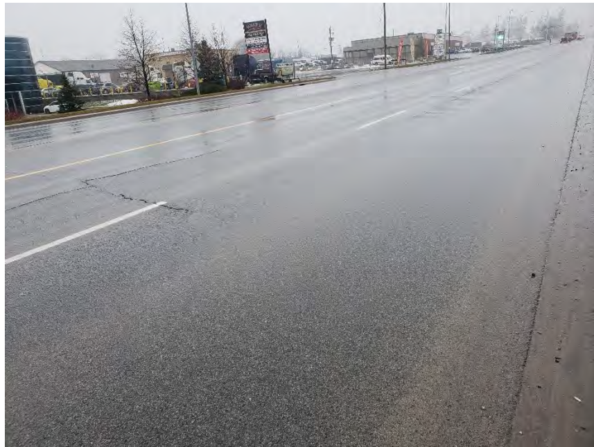
Photograph 22 – Region Road 25, Northbound, 90m north of Peddie Road, looking north, showing slight to moderate longitudinal and transverse cracking.
