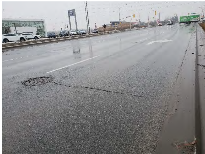
Photograph 10 – Region Road 25, Northbound, 70m south of James Snow Parkway North, looking north, showing slight to moderate transverse cracking around the maintenance hole.
