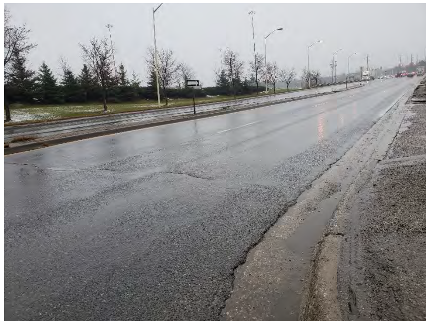
Photograph 6 – Region Road 25, Southbound, 10m South of Chisholm Drive, looking south, showing slight transverse cracking, slight ravelling and slight pavement edge cracking
