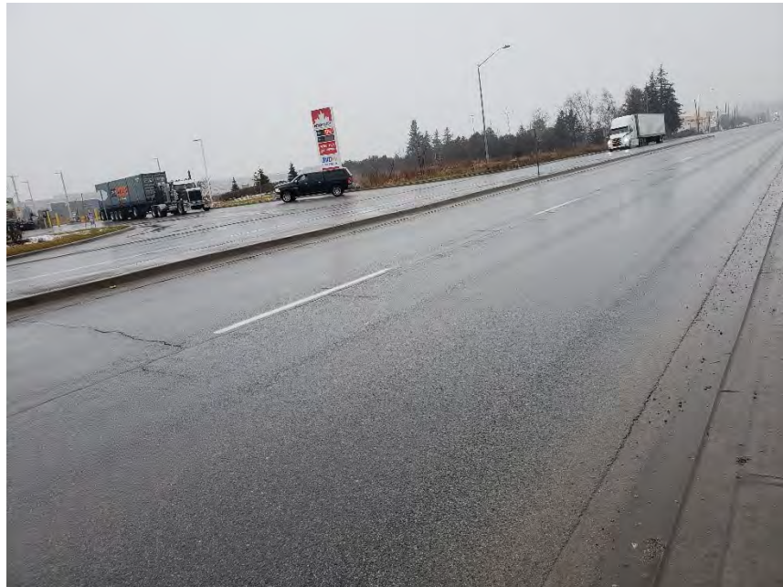
Photograph 12 – Region Road 25, Northbound, 50m north of James Snow Parkway, looking north, showing slight to moderate longitudinal and transverse cracking.
