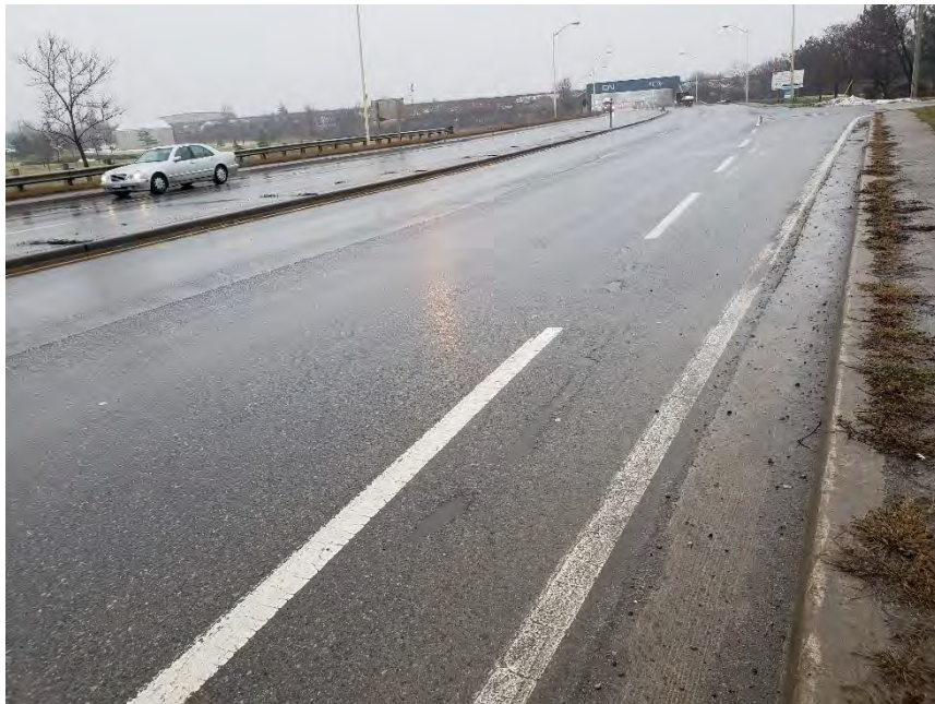
Photograph 4 – Region Road 25, Southbound, 20m South of Market Drive, looking south, showing slight longitudinal cracking.
