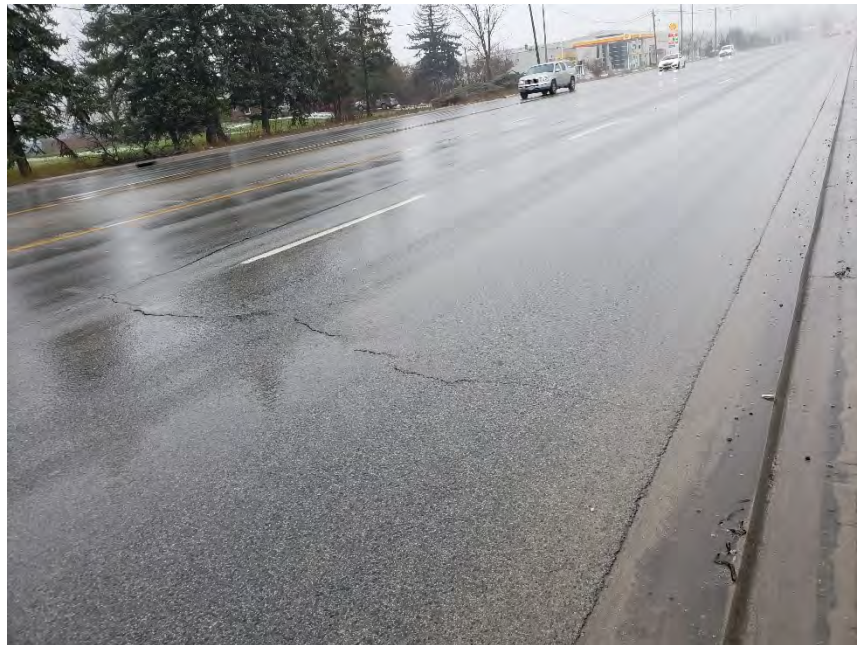
Photograph 16 – Region Road 25, Northbound, 200m north of James Snow Parkway, looking north, showing slight longitudinal and transverse cracking.
