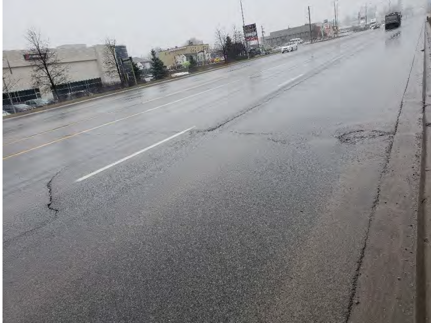
Photograph 21 – Region Road 25, Northbound, 70m north of Peddie Road, looking north, showing slight to moderate longitudinal and transverse cracking.
