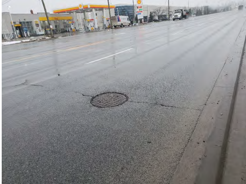
Photograph 17 – Region Road 25, Northbound, 300m south of Peddie Road, looking north, showing slight transverse cracking around the maintenance hole.
