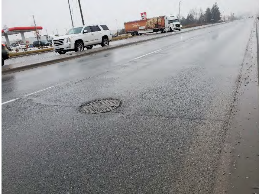
Photograph 11 – Region Road 25, Northbound, 15m north of James Snow Parkway, looking north, showing slight longitudinal cracking and slight transverse cracking around the maintenance hole.
