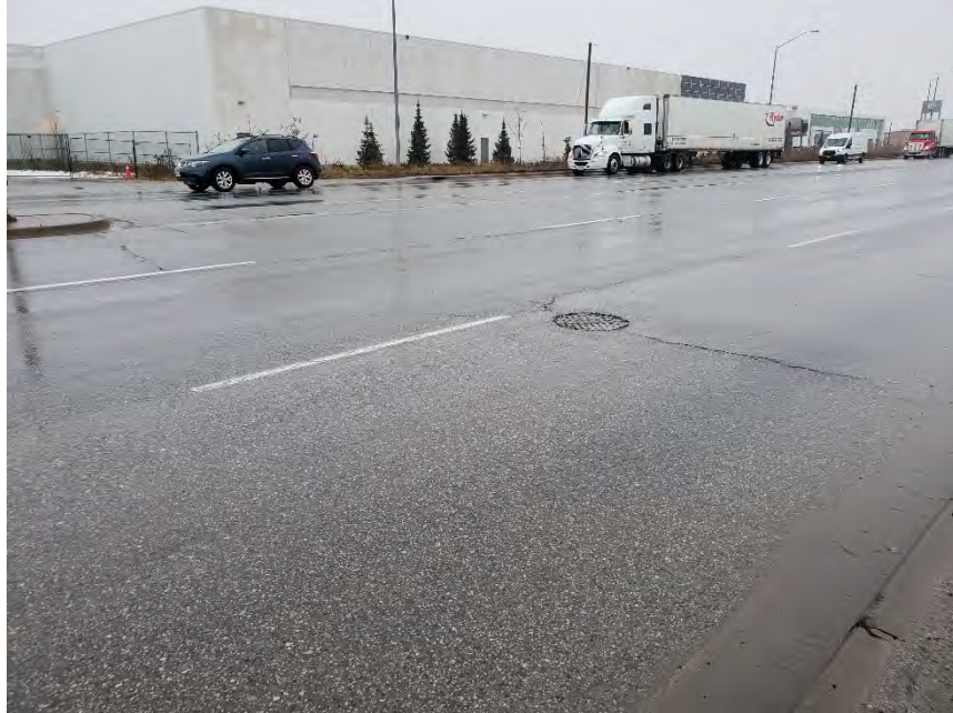
Photograph 7 – Region Road 25, Northbound, 15m north of Highpoint Drive, looking north, showing slight to moderate longitudinal and transverse cracking and slight random cracking around the maintenance hole.
