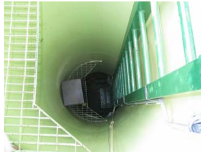
Access to pump chamber
