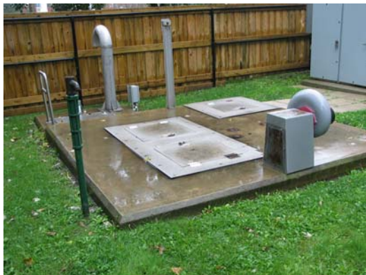
External access to pump chamber and wet well
