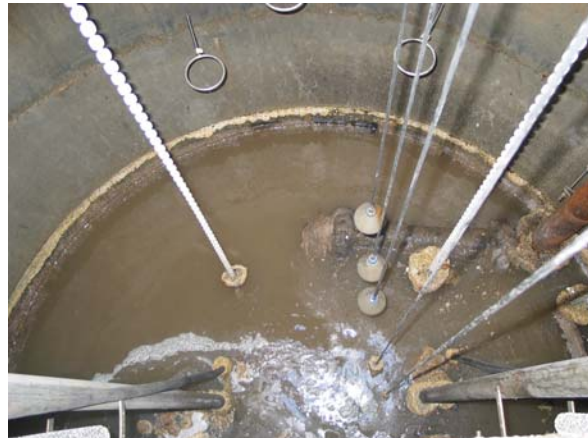
Submersible pumps in wet well
