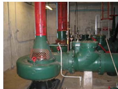
Pump & discharge piping – 2 nd level below grade in drywell
