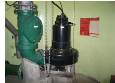
Pump and discharge piping
