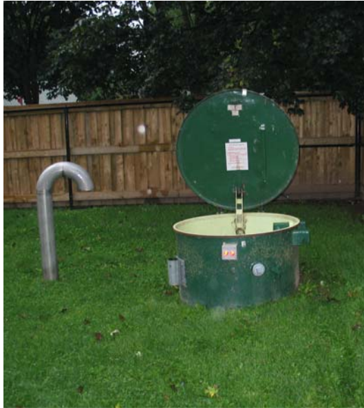
External access to pump chamber and wet well
