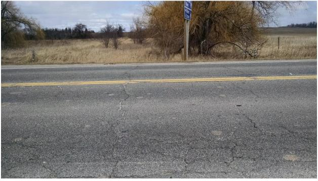
Photograph 7 – Deteriorated Pavement Condition South of 10 Side Road
