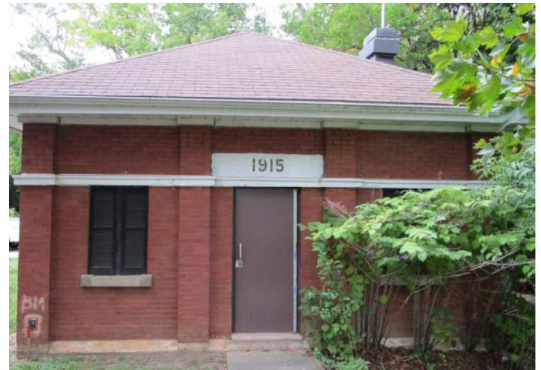
Existing Junction WWPS
