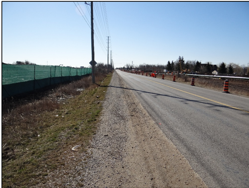
Figure 19: Narrow Gravel Shoulders on Ninth Line south of Burnhamthorpe Road
