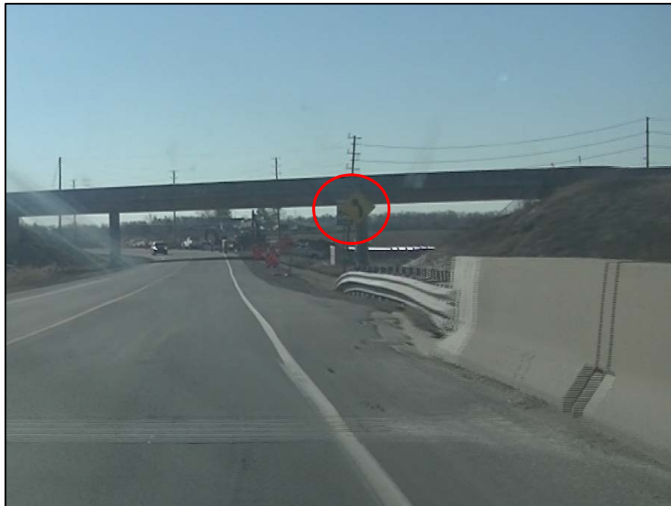
Figure 15: Curve Warning Sign Blocking Speed Limit Sign (Southbound)
