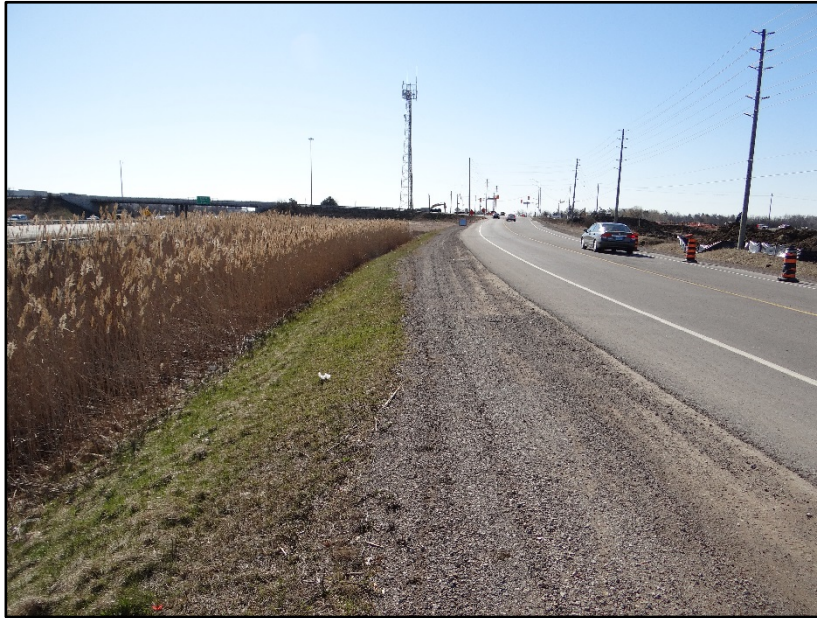
Figure 20: Paved and Gravel Shoulder on Ninth Line North of Burnhamthorpe Road
