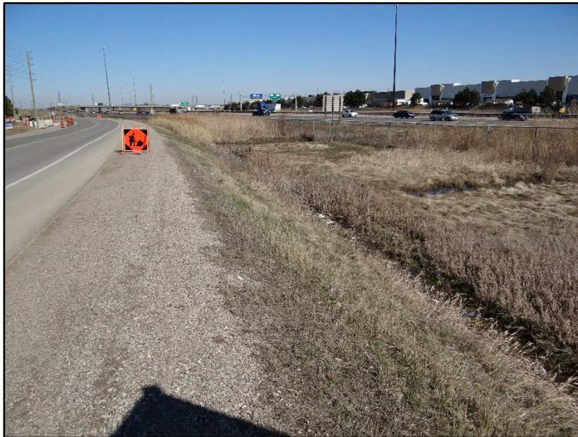
Figure 21: Typical Side Slope on Ninth Line north of Burnhamthorpe Road
