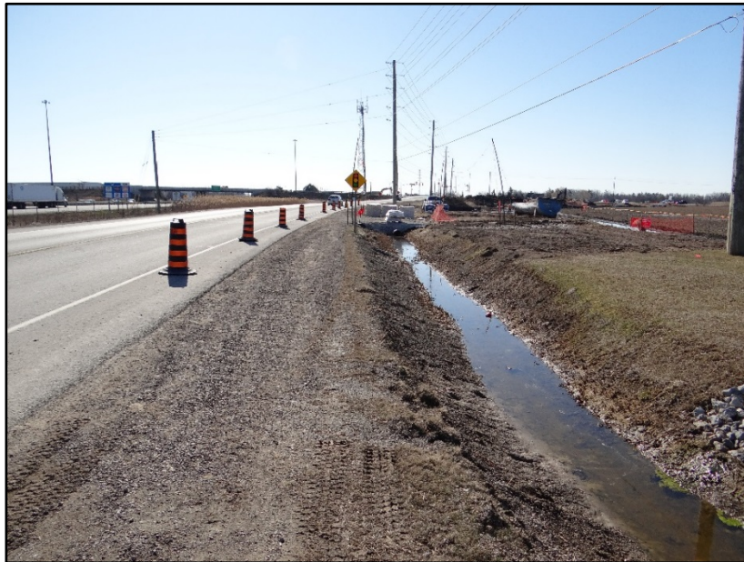
Figure 23: Culvert on West Side of Ninth Line north of Burnhamthorpe Road
