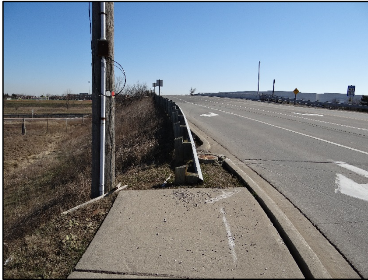
Figure 18: Pedestrian Facility along East Leg of Intersection (Burnhamthorpe Road West)
