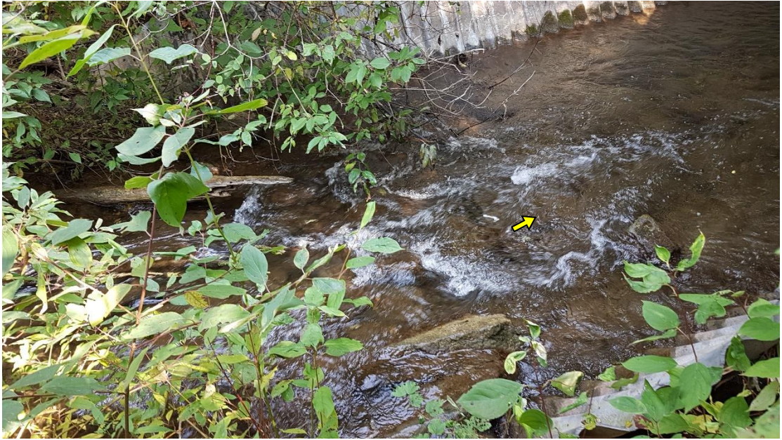
The culverts were slightly embedded into the riverbed.
