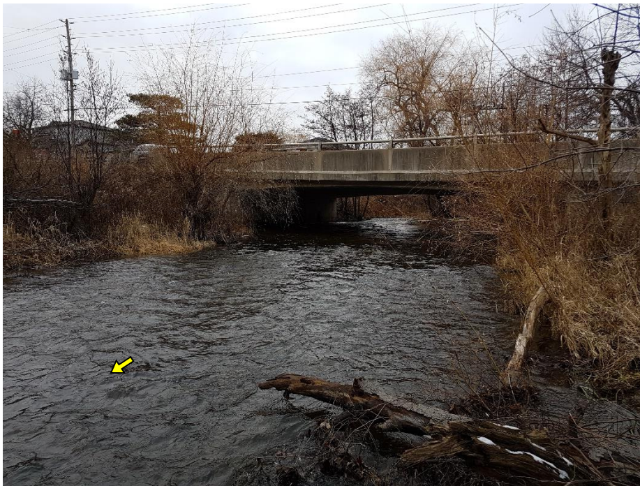
The Steeles Avenue crossing was undersized relative to the channel. The channel wetted width extended the full span of the crossing.
