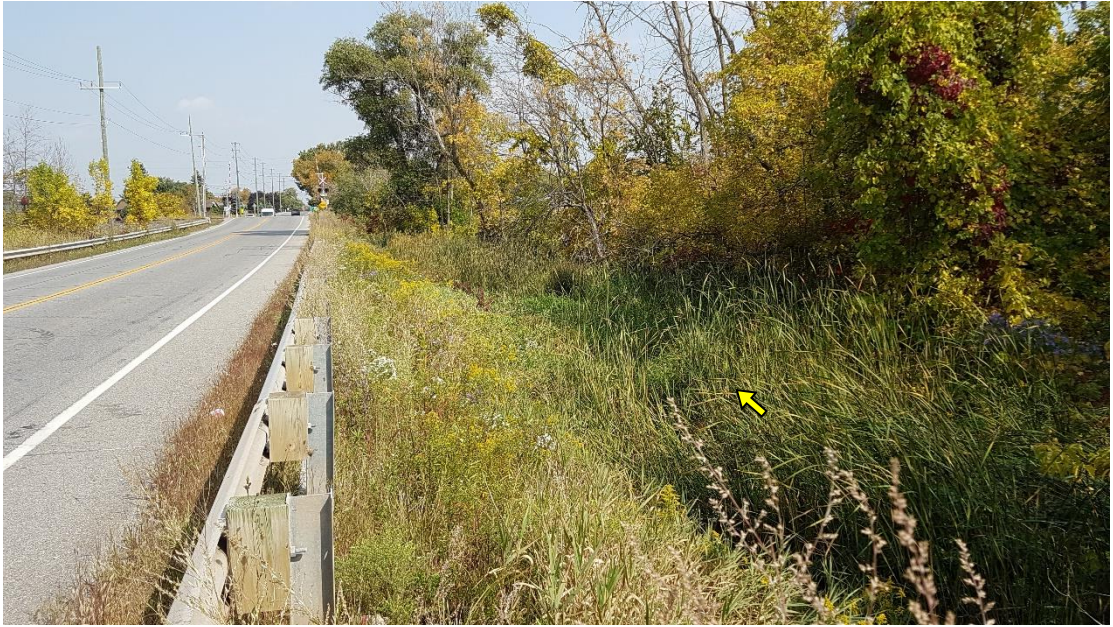
NW-1-E consisted of a 2.5 m wide, well-vegetated swale, which extended from the adjacent farm field and followed the Steeles Avenue embankment.
