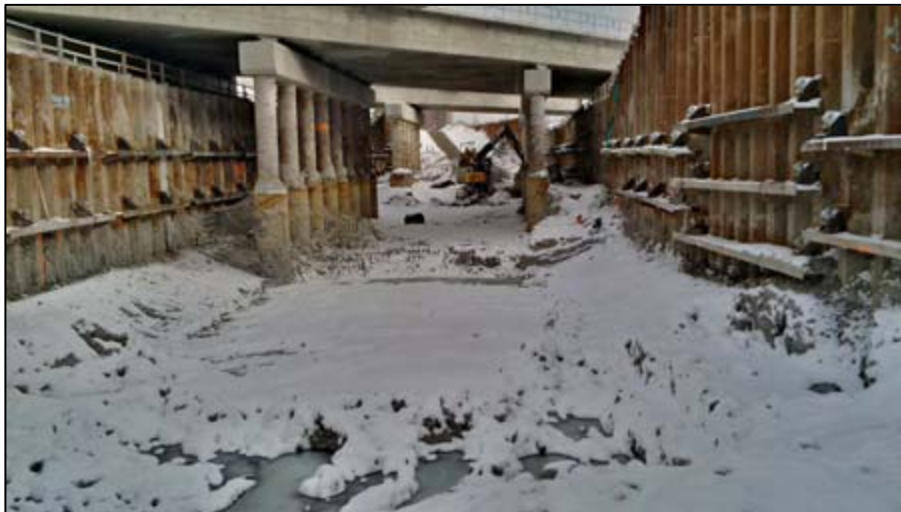
Figure 1: Denison Road Underpass.
