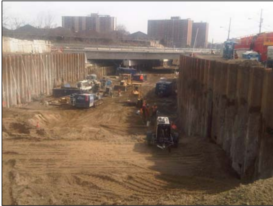
Figure 2: Denison Road Underpass.
