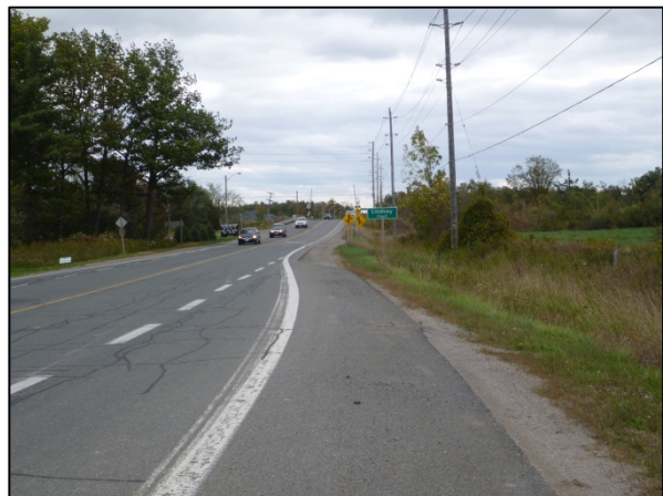
Plate 12: Field conditions within the study corridor, facing southeast. Note disturbance within the ROW, and areas of archaeological potential outside the ROW.
