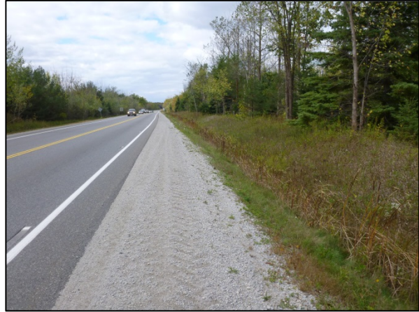
Plate 2: Field conditions within the study corridor, facing west. Note disturbance within the ROW, and areas of archaeological potential outside the ROW.
