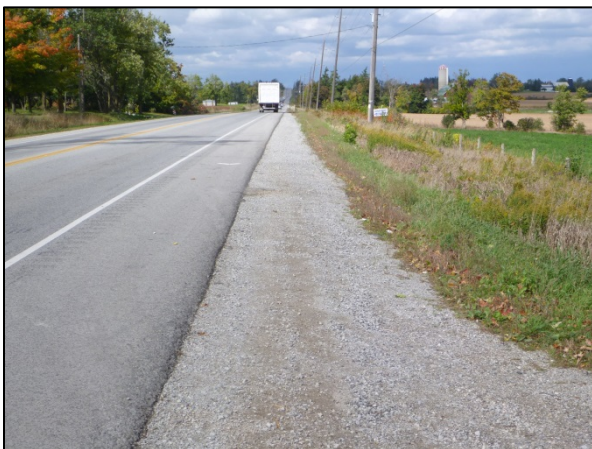
Plate 5: Field conditions within the study corridor, facing northwest. Note disturbance within the ROW, and areas of archaeological potential outside the ROW.
