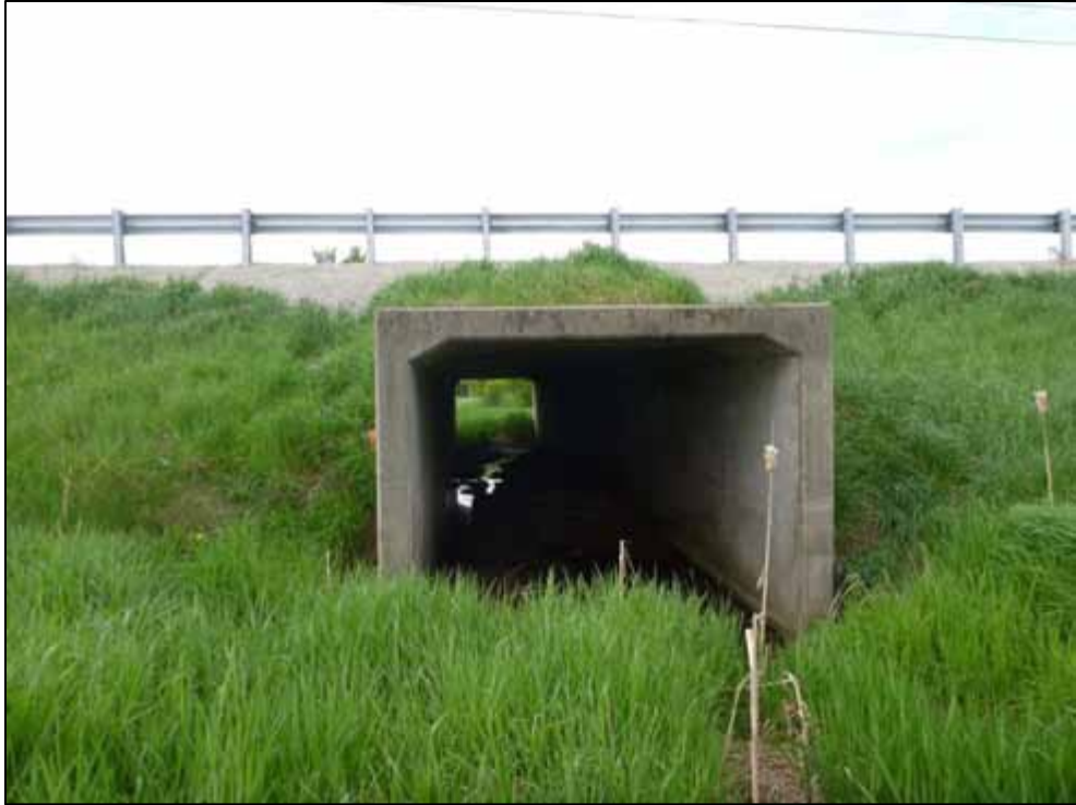
Photo 1: Culvert C1, downstream face (looking west)
