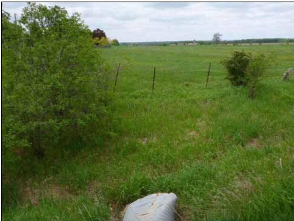
Photo 48: Culvert C12, upstream channel (looking west)
