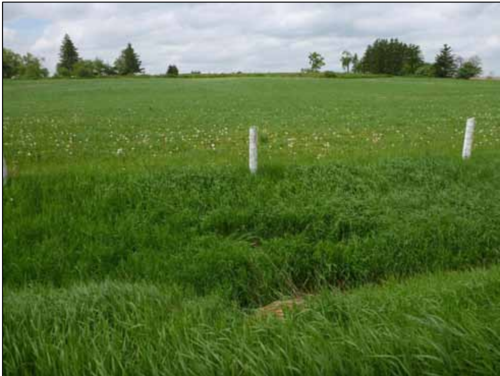
Photo 26: Culvert C7, downstream channel (looking east)
