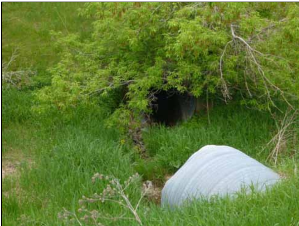
Photo 74: Culvert C18, downstream channel (looking east towards C16)
