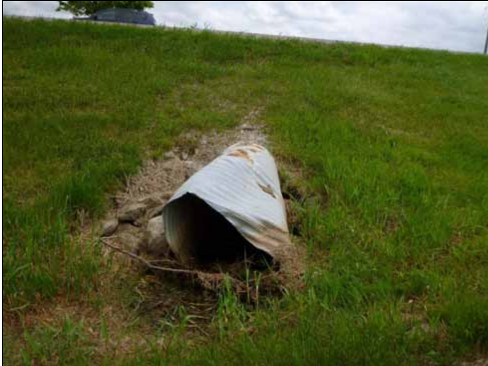
Photo 39: Culvert C10, upstream face (looking east)
