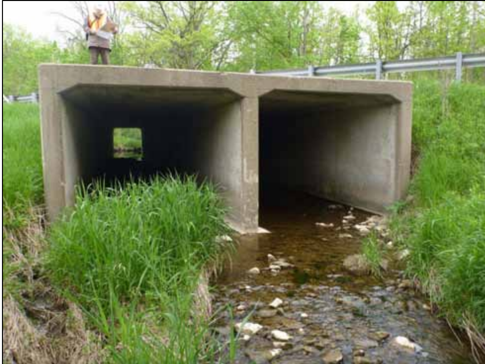
Photo 5: Culvert C2, downstream face (looking north)
