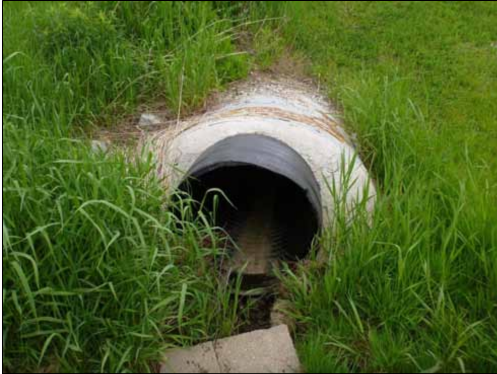
Photo 43: Culvert C11, upstream face (looking east)
