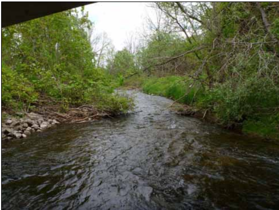
Photo 50: Bridge B1, downstream channel (looking east)
