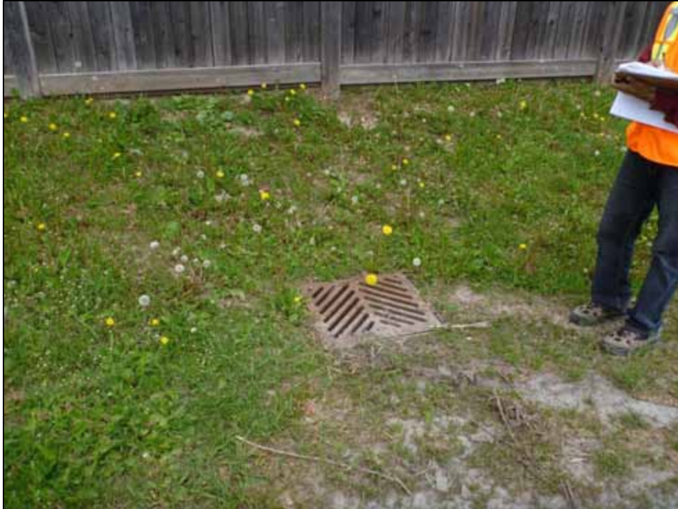
Photo 65: Storm Sewer S1, downstream manhole
