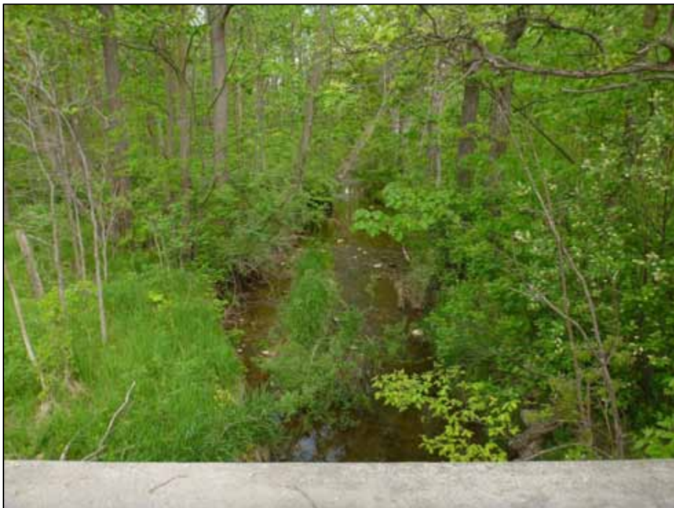
Photo 8: Culvert C2, upstream channel (looking north)
