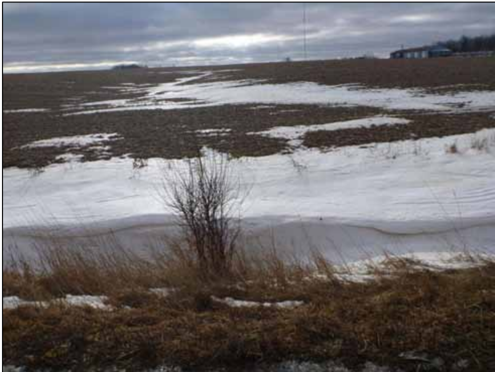
Photo 20: Culvert C5, upstream channel (looking west)
