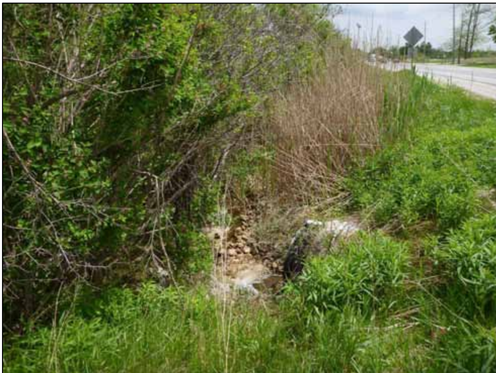
Photo 58: Culvert C14, downstream channel (looking south)
