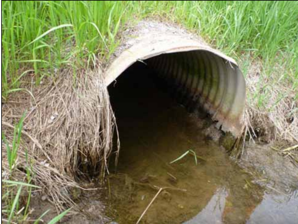
Photo 37: Culvert C10, downstream face (looking west)
