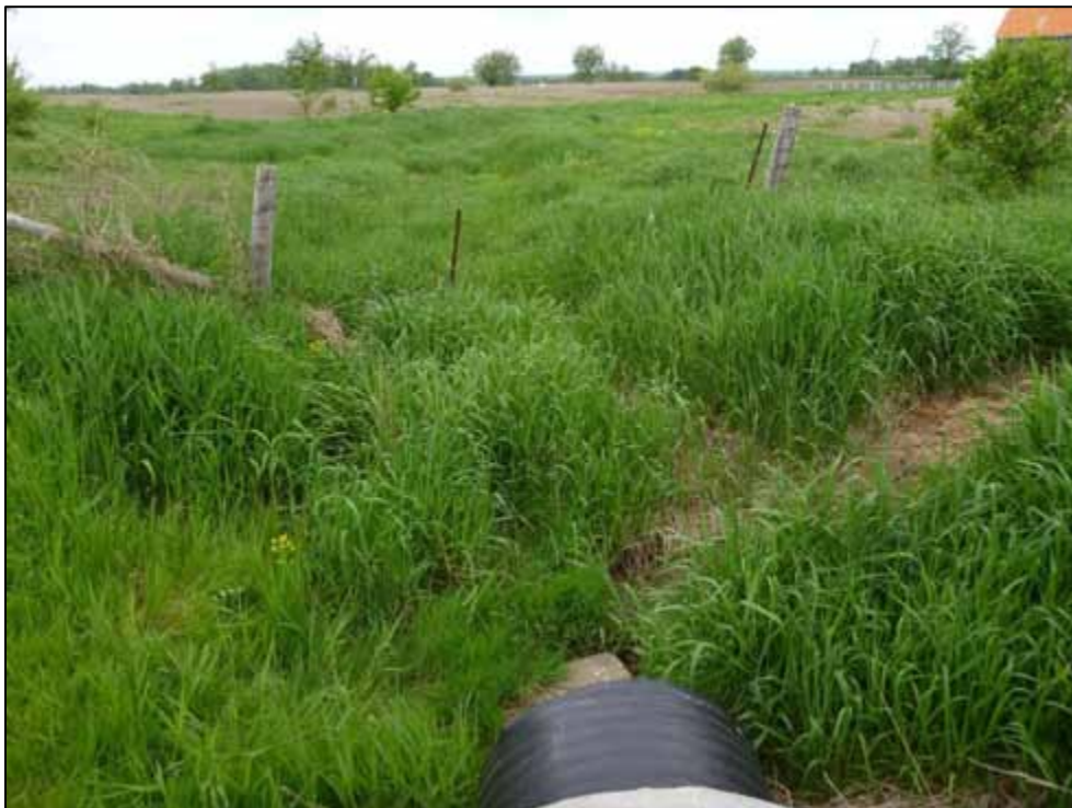
Photo 44: Culvert C11, upstream channel (looking west)
