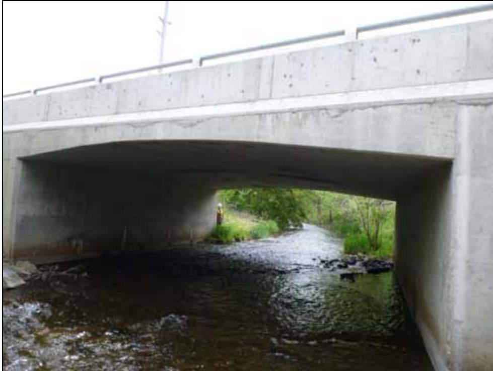
Photo 49: Bridge B1, downstream face (looking west)
