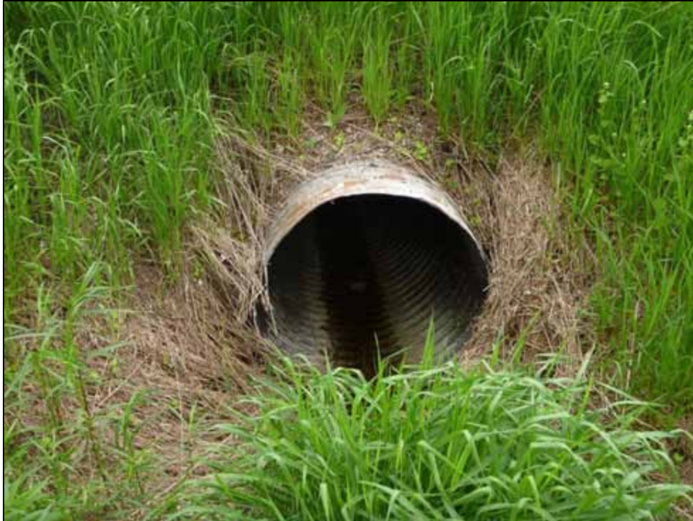
Photo 23: Culvert C6, upstream face (looking east)
