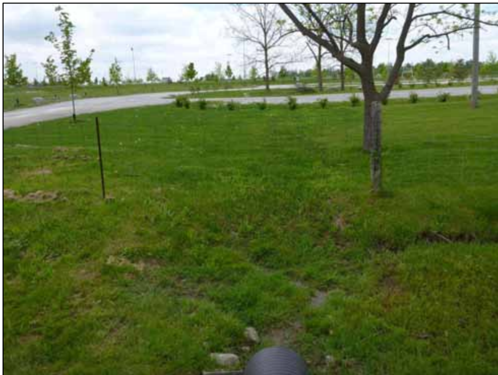
Photo 56: Culvert C13, upstream channel (looking west)
