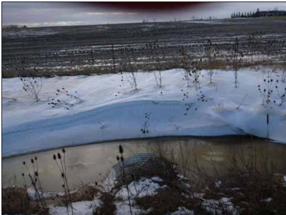
Photo 36: Culvert C9, upstream channel (looking west)
