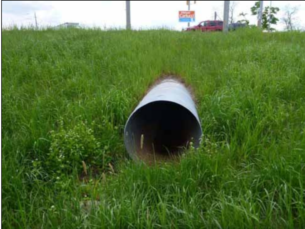
Photo 75: Culvert C17, downstream face (looking west)
