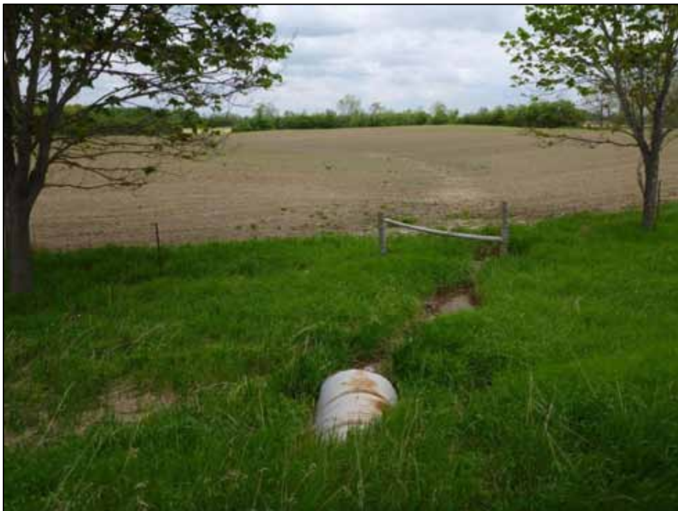
Photo 46: Culvert C12, downstream channel (looking east)
