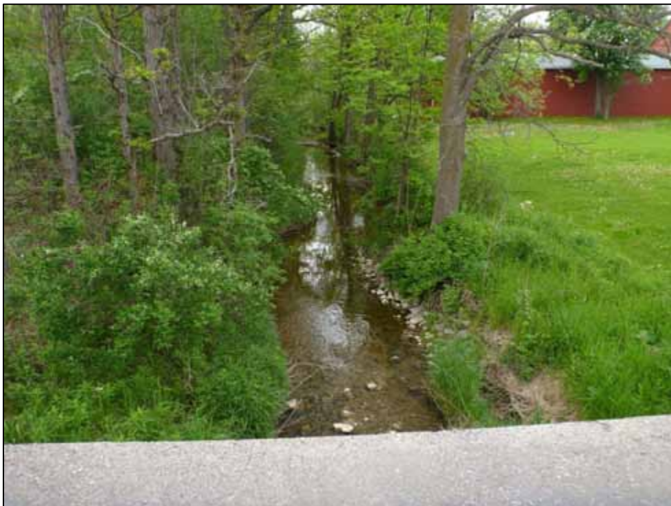
Photo 6: Culvert C2, downstream channel (looking south)
