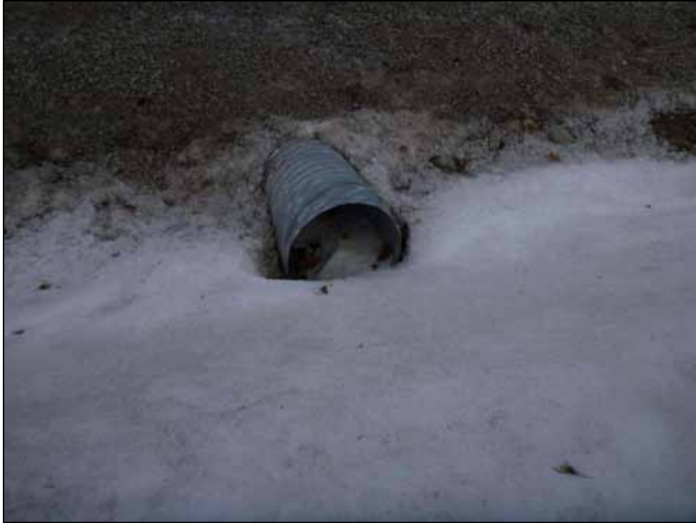
Photo 15: Culvert C4, upstream face (looking east)
