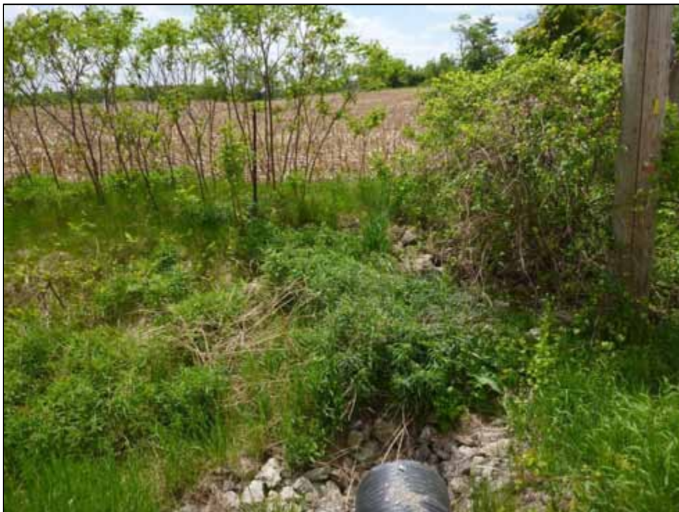
Photo 68: Storm Sewer S1, upstream channel (looking west)
