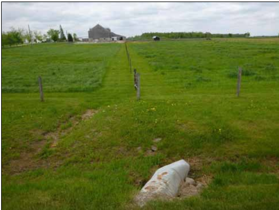
Photo 40: Culvert C10, upstream channel (looking west)
