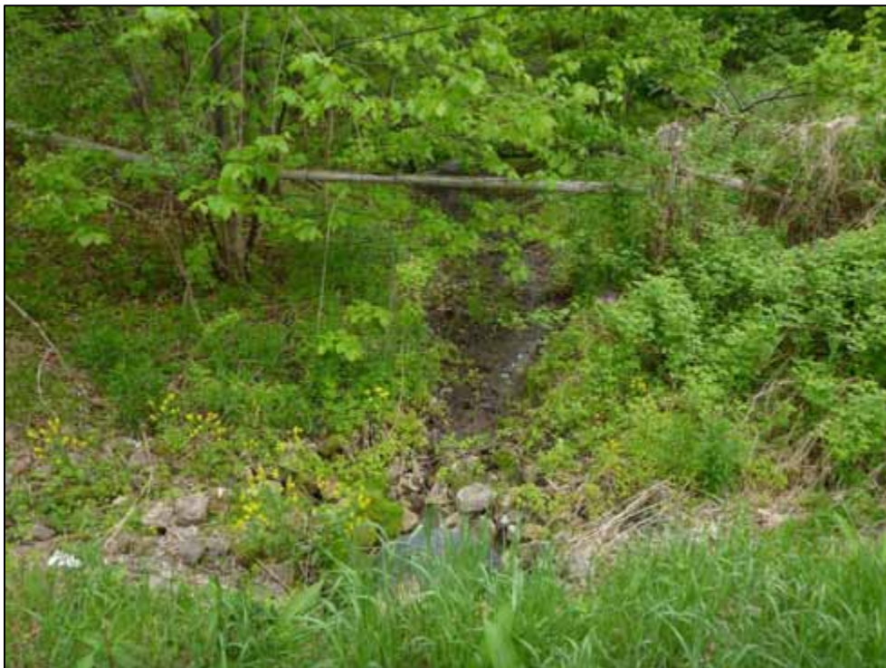
Photo 64: Culvert C15, upstream channel (looking west)
