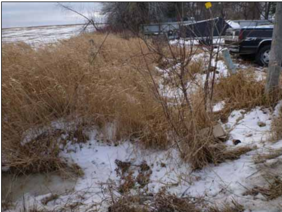
Photo 32: Culvert C8, upstream channel (looking west)
