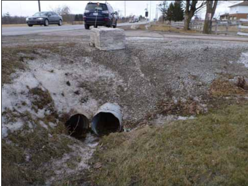
Photo 11: Culvert C3, upstream face (looking west)
