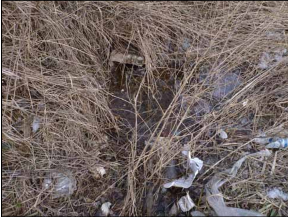
Photo 9: Culvert C3, downstream face (looking east)
