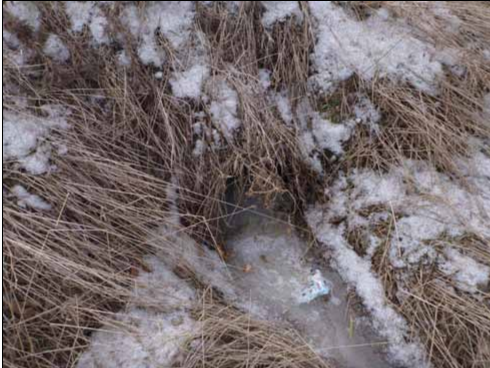
Photo 17: Culvert C5, downstream face (looking west)
