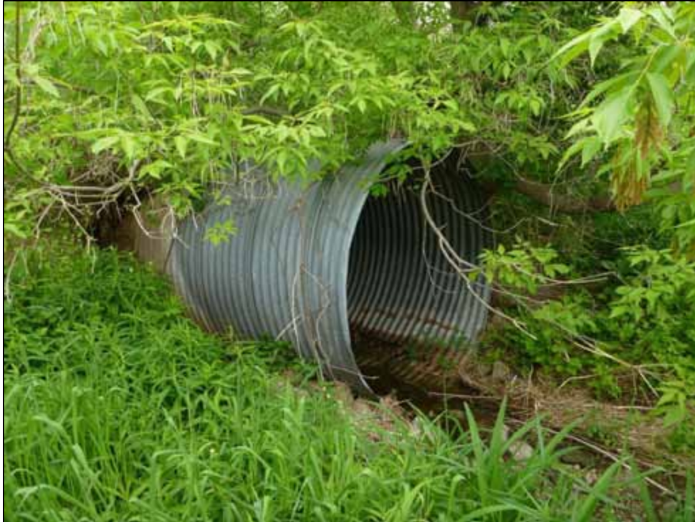
Photo 71: Culvert C16, upstream face (looking south-east)
