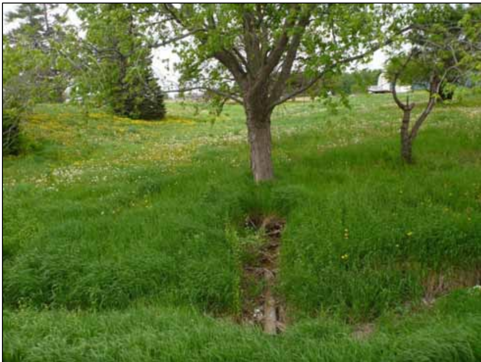
Photo 24: Culvert C6, upstream channel (looking west)
