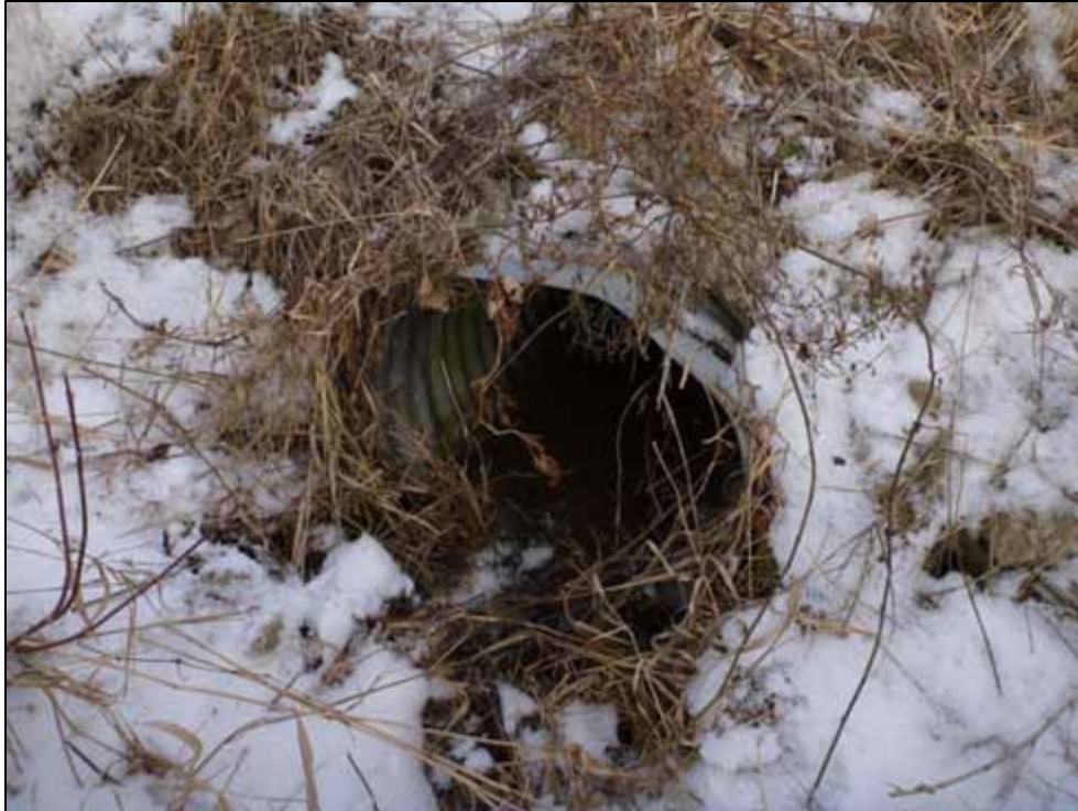
Photo 31: Culvert C8, upstream face (looking east)
