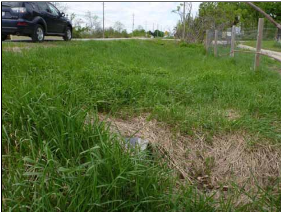
Photo 54: Culvert C13, downstream channel (looking north)
