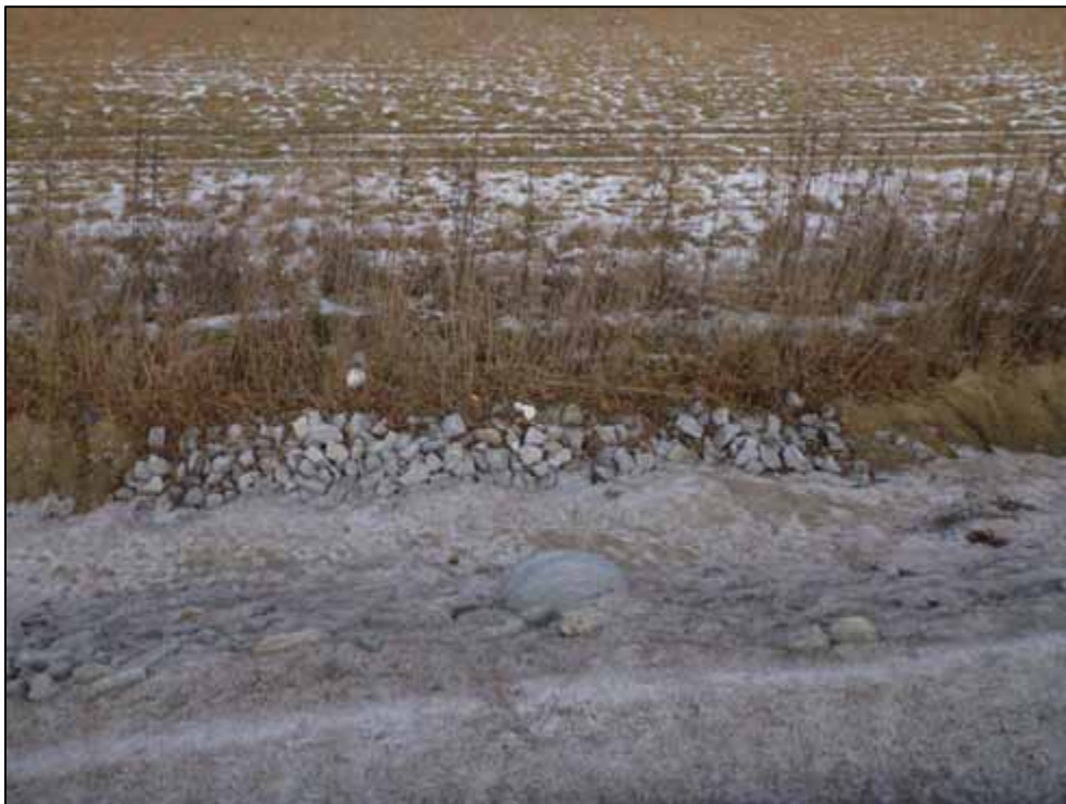
Photo 14: Culvert C4, downstream channel (looking east)
