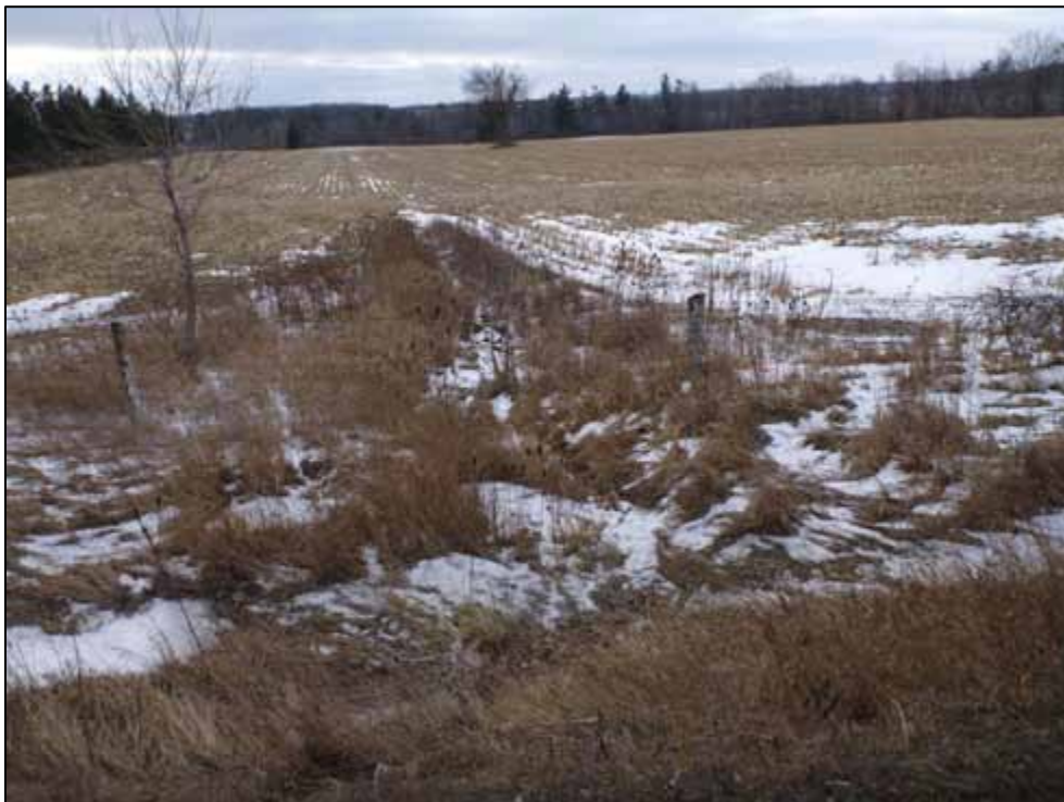
Photo 10: Culvert C3, downstream channel (looking west)
