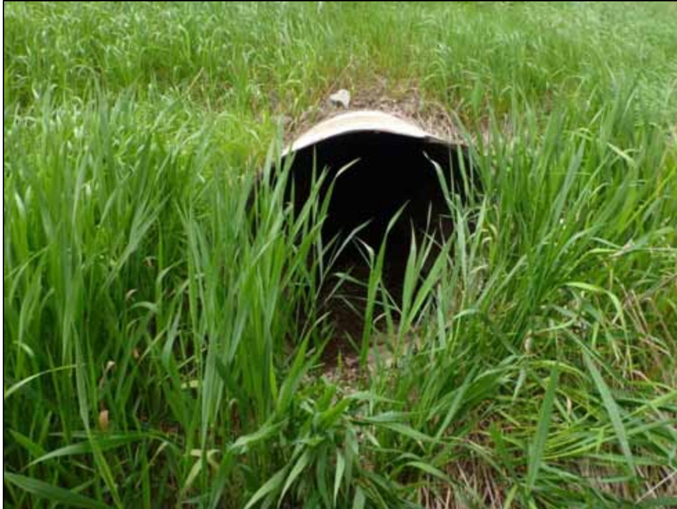
Photo 45: Culvert C12, downstream face (looking west)
