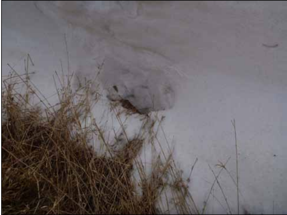
Photo 19: Culvert C5, upstream face (looking east)
