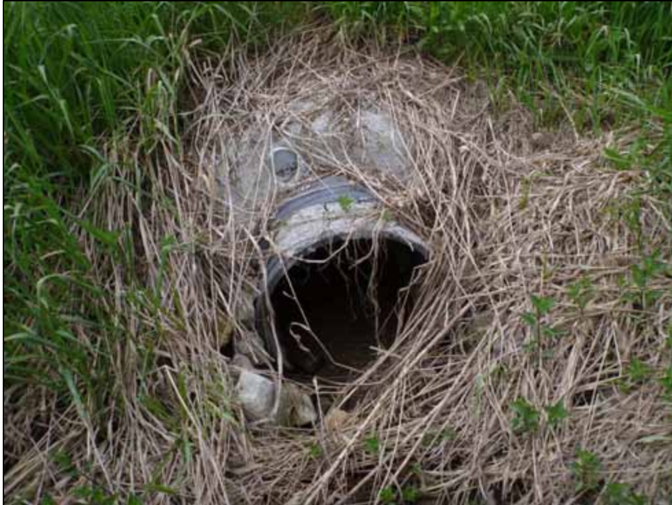
Photo 53: Culvert C13, downstream face (looking west)
