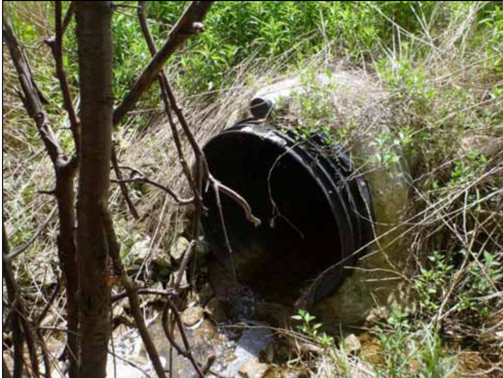
Photo 57: Culvert C14, downstream face (looking west)
