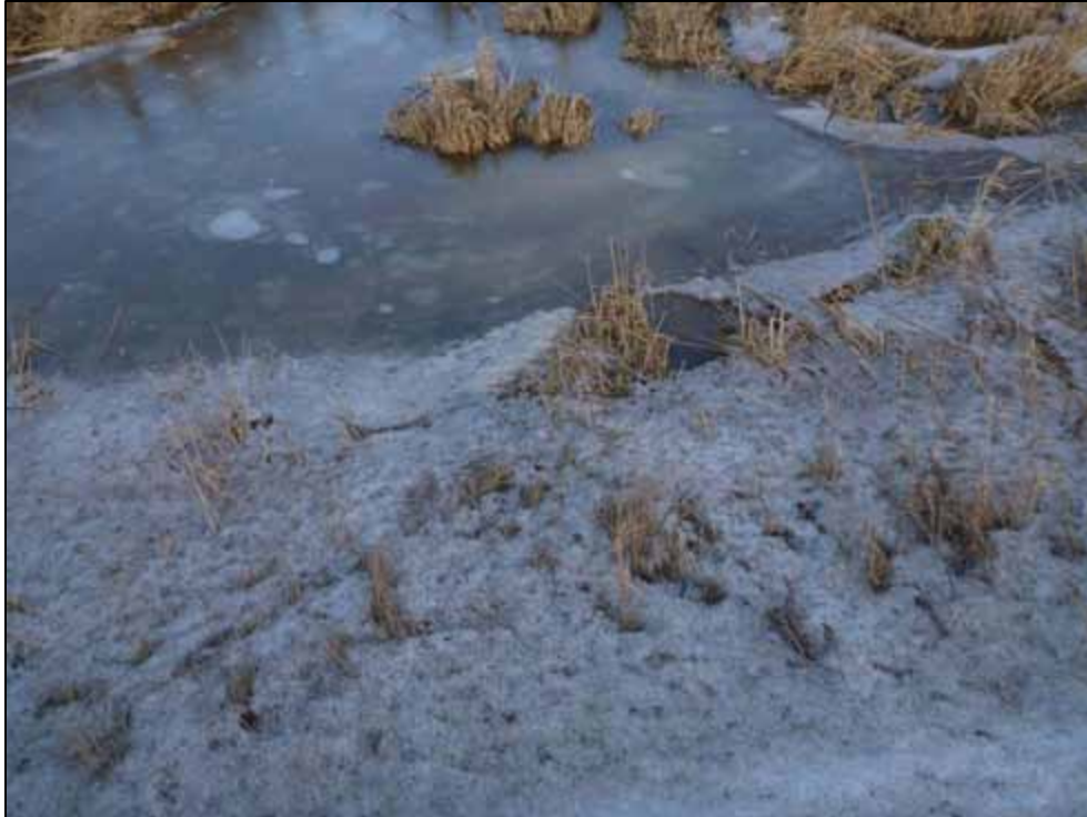
Photo 33: Culvert C9, downstream face (looking west), submerged
