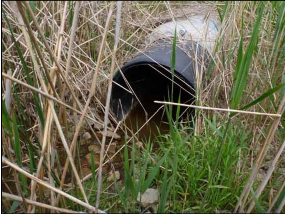
Photo 59: Culvert C14, upstream face (looking east)
