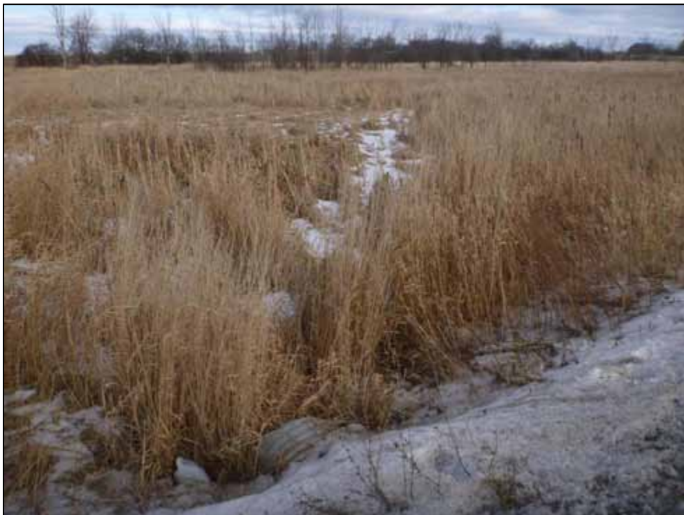
Photo 30: Culvert C8, downstream channel (looking east)
