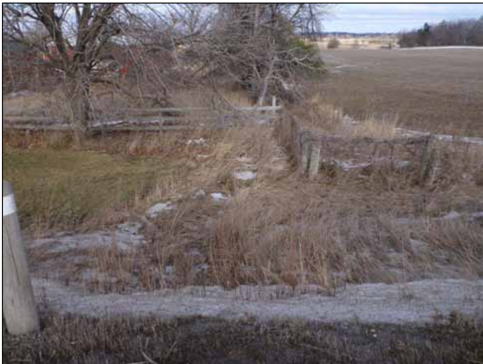
Photo 18: Culvert C5, downstream channel (looking east)
