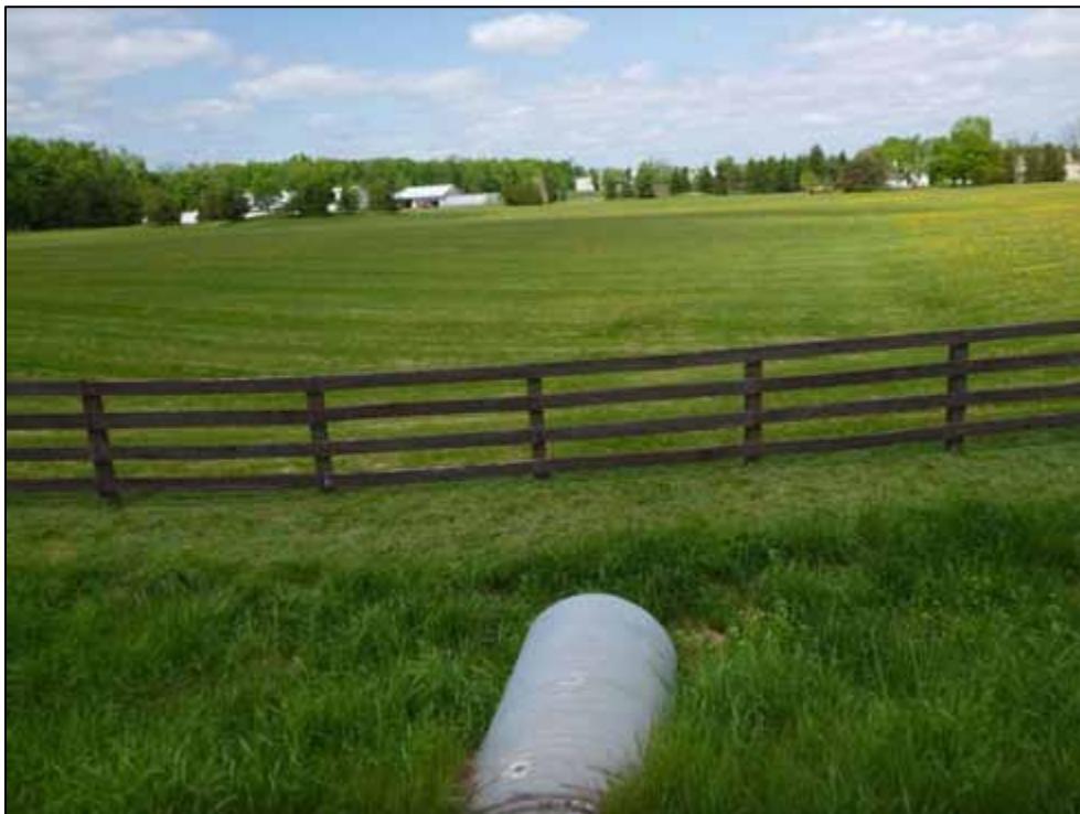
Photo 76: Culvert C17, downstream channel (looking east)
