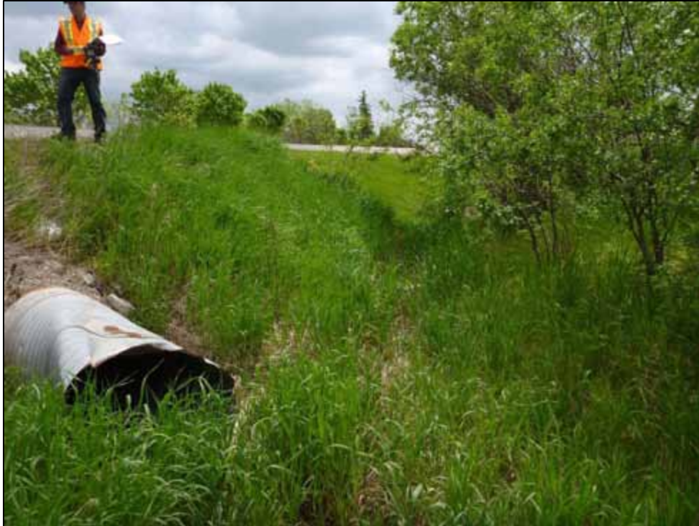
Photo 47: Culvert C12, upstream face (looking east)
