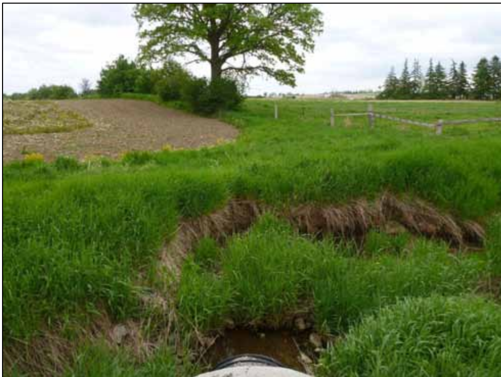
Photo 42: Culvert C11, downstream channel (looking east)
