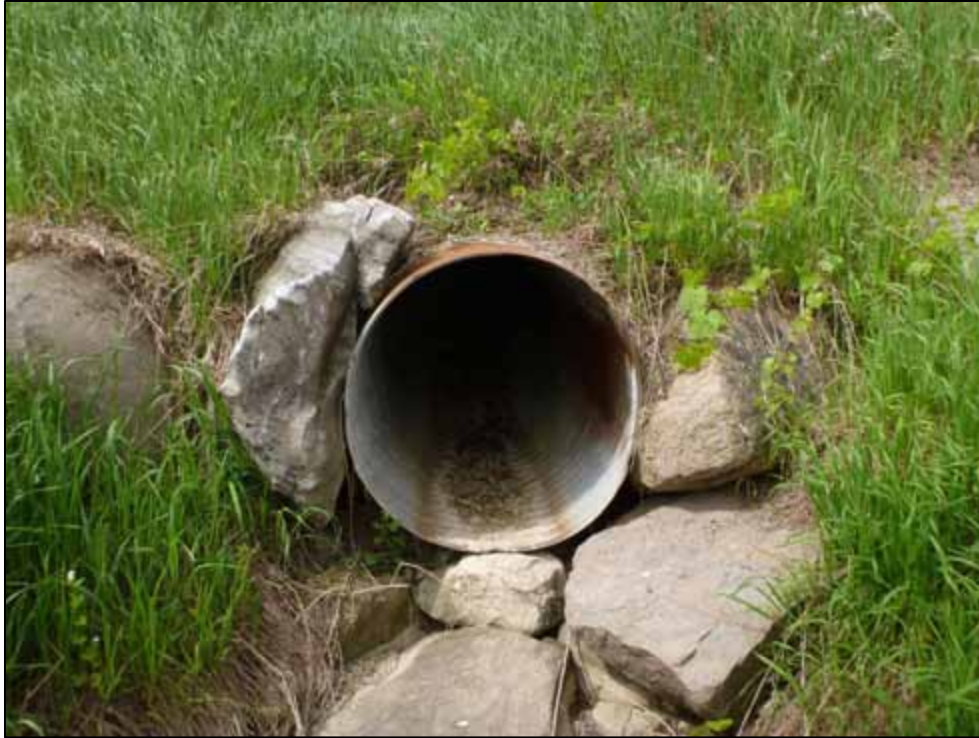
Photo 21: Culvert C6, downstream face (looking west)
