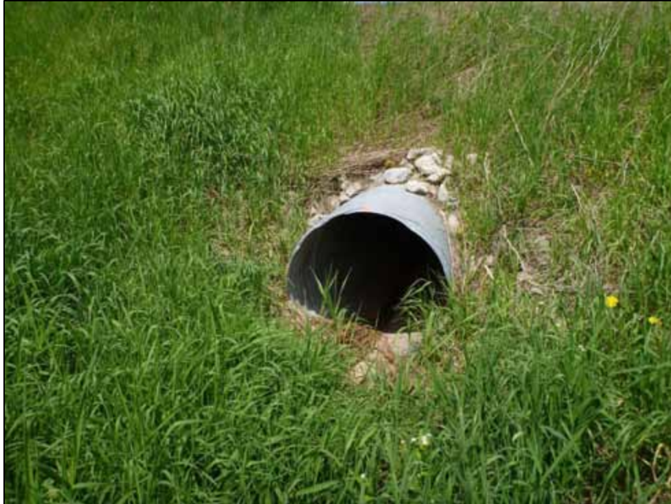
Photo 77: Culvert C17, upstream face (looking east)
