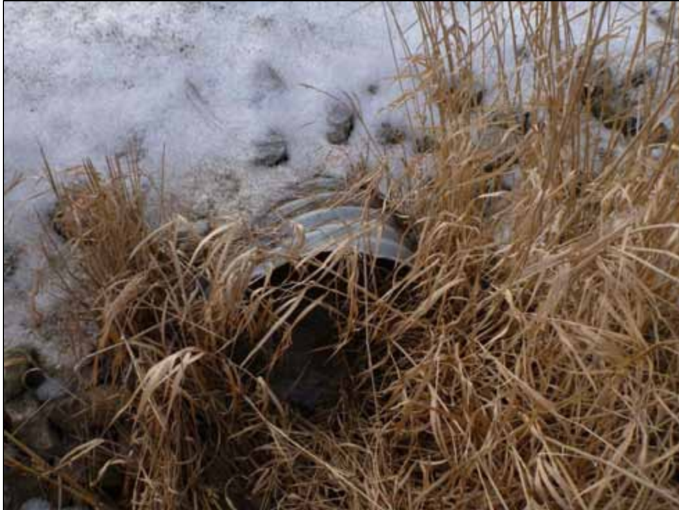
Photo 29: Culvert C8, downstream face (looking west)
