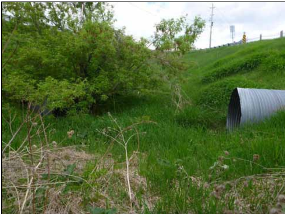
Photo 72: Culvert C16, upstream channel (looking south with C18 on the right)
