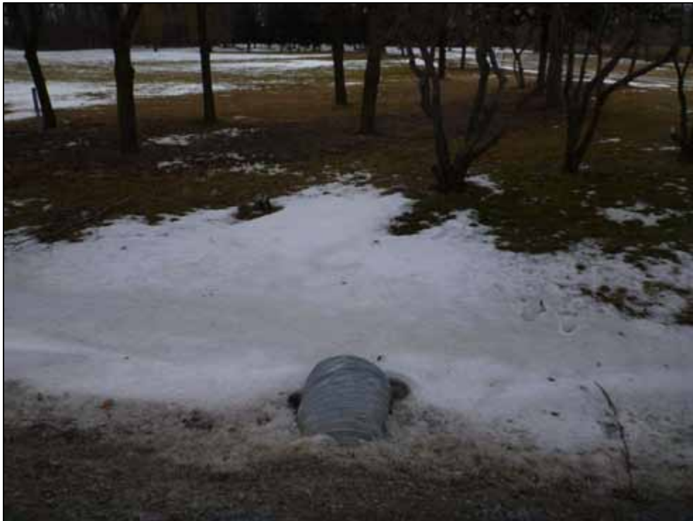
Photo 16: Culvert C4, upstream channel (looking west)
