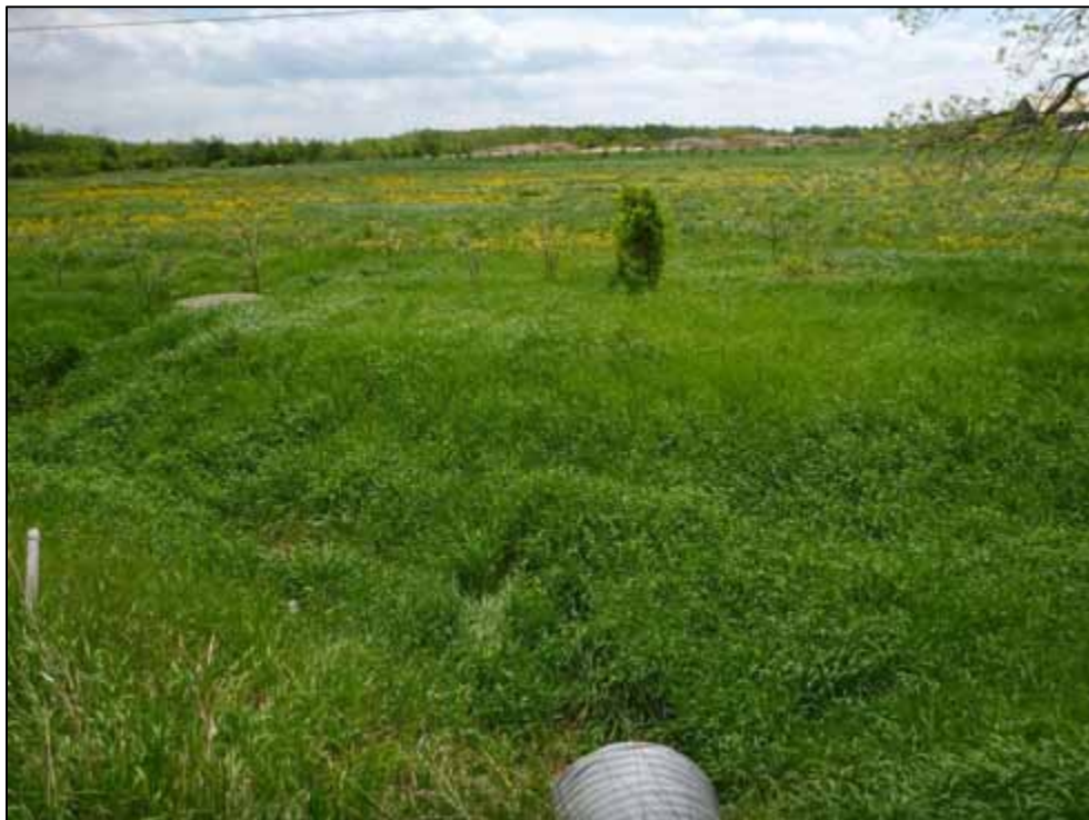
Photo 78: Culvert C17, upstream channel (looking west)
