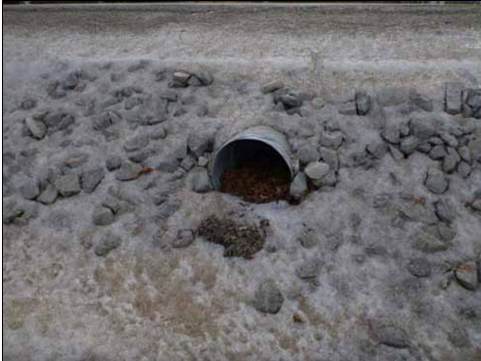
Photo 13: Culvert C4, downstream face (looking west)
