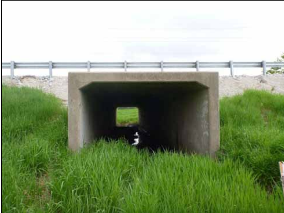
Photo 3: Culvert C1, upstream face (looking east)
