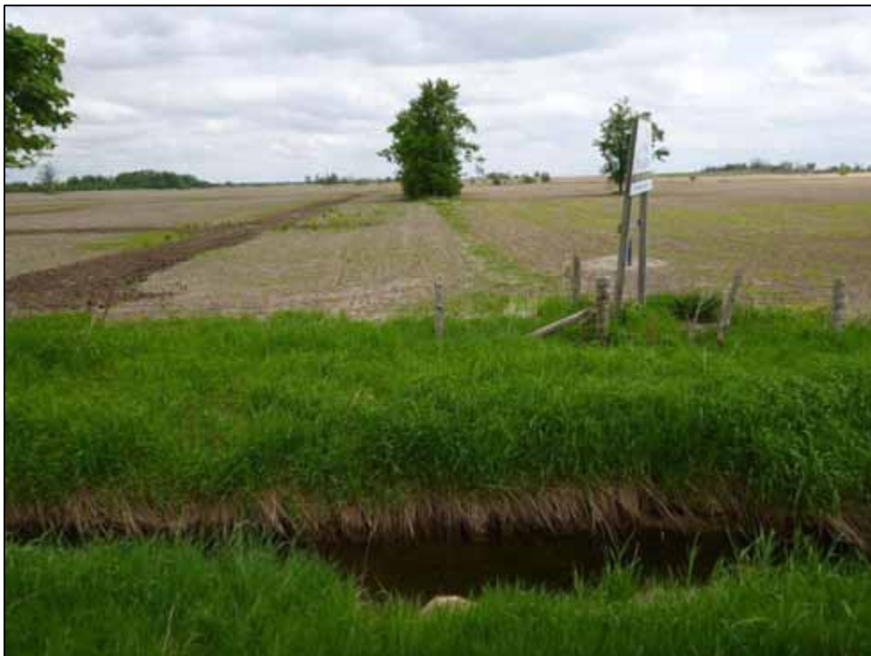
Photo 38: Culvert C10, downstream channel (looking east)
