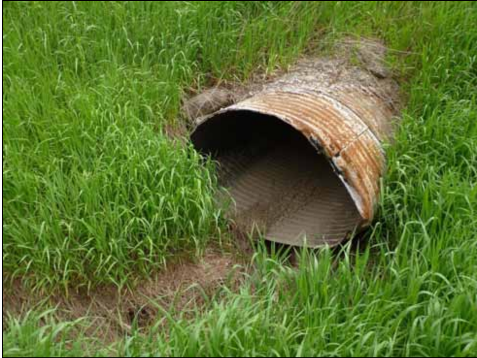
Photo 25: Culvert C7, downstream face (looking west)
