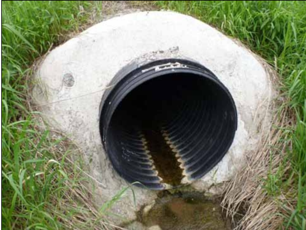
Photo 41: Culvert C11, downstream face (looking west)
