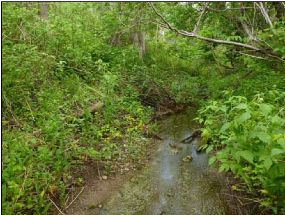
Photo 70: Culvert C16, downstream channel (looking east)
