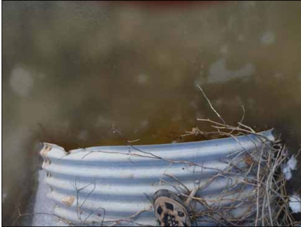
Photo 35: Culvert C9, upstream face (looking east)
