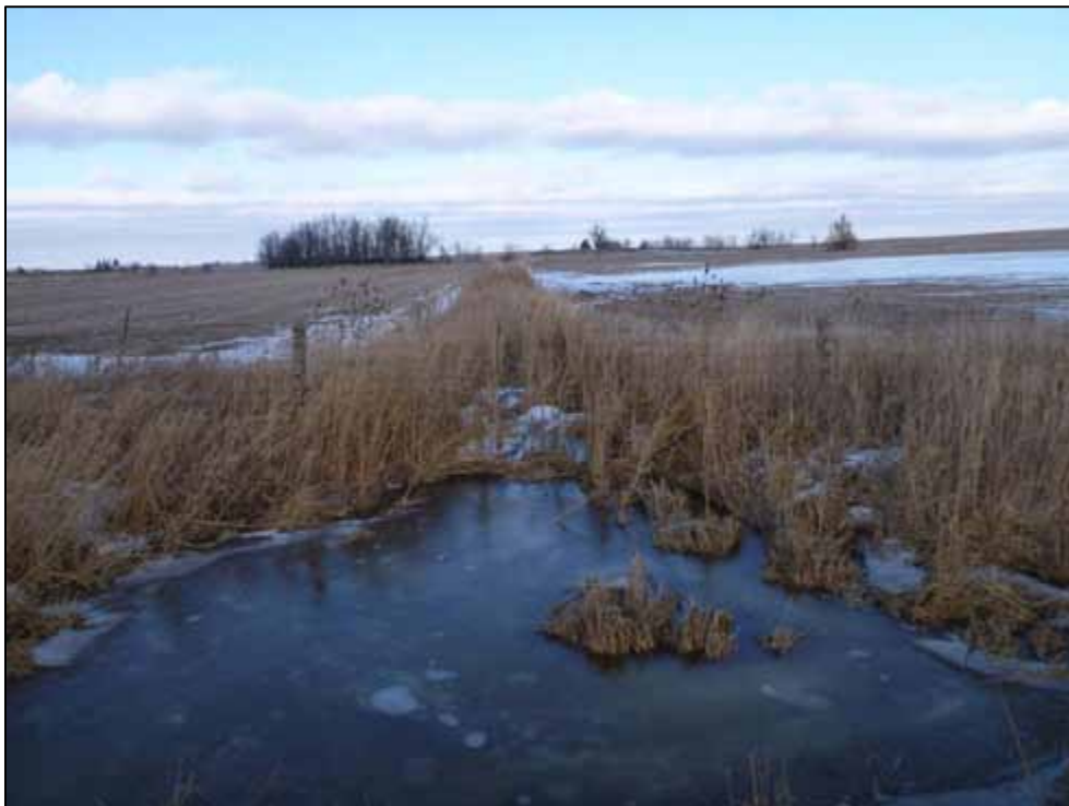
Photo 34: Culvert C9, downstream channel (looking east)
