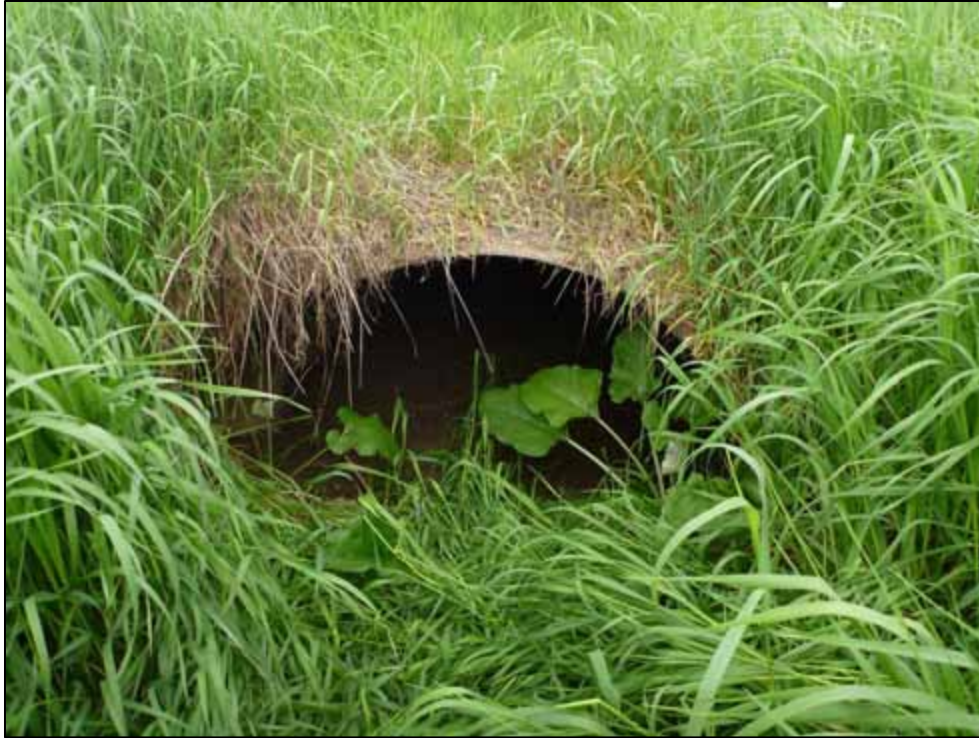
Photo 27: Culvert C7, upstream face (looking east)
