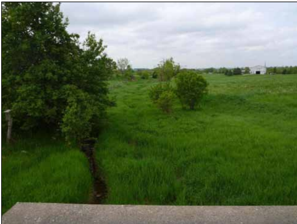
Photo 4: Culvert C1, upstream channel (looking west)
