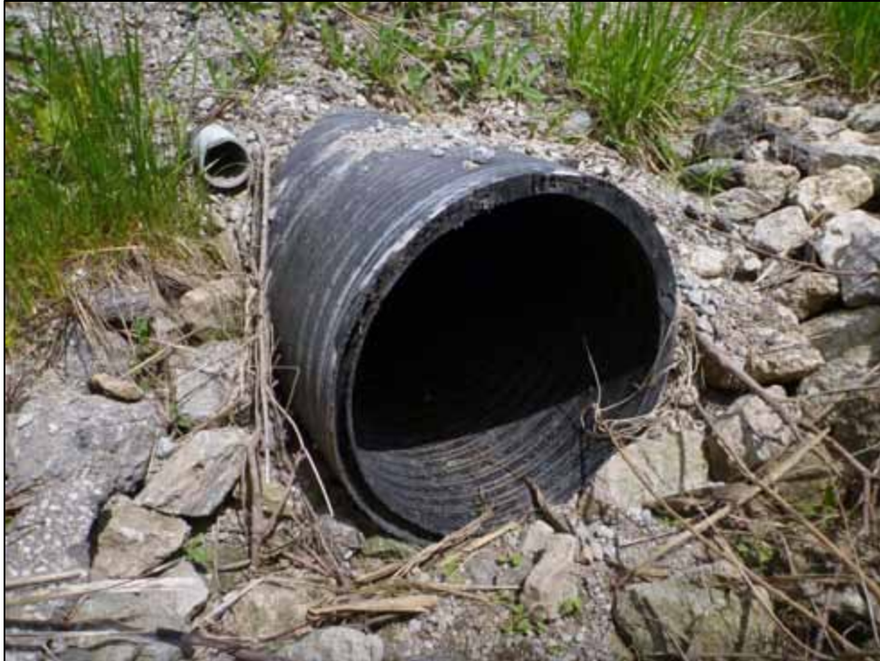
Photo 67: Storm Sewer S1, upstream face (looking east)
