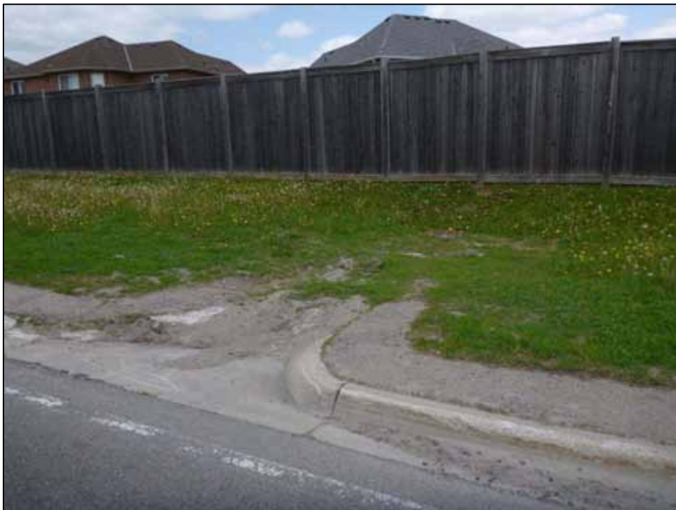
Photo 66: Storm Sewer S1, downstream manhole (looking east)
