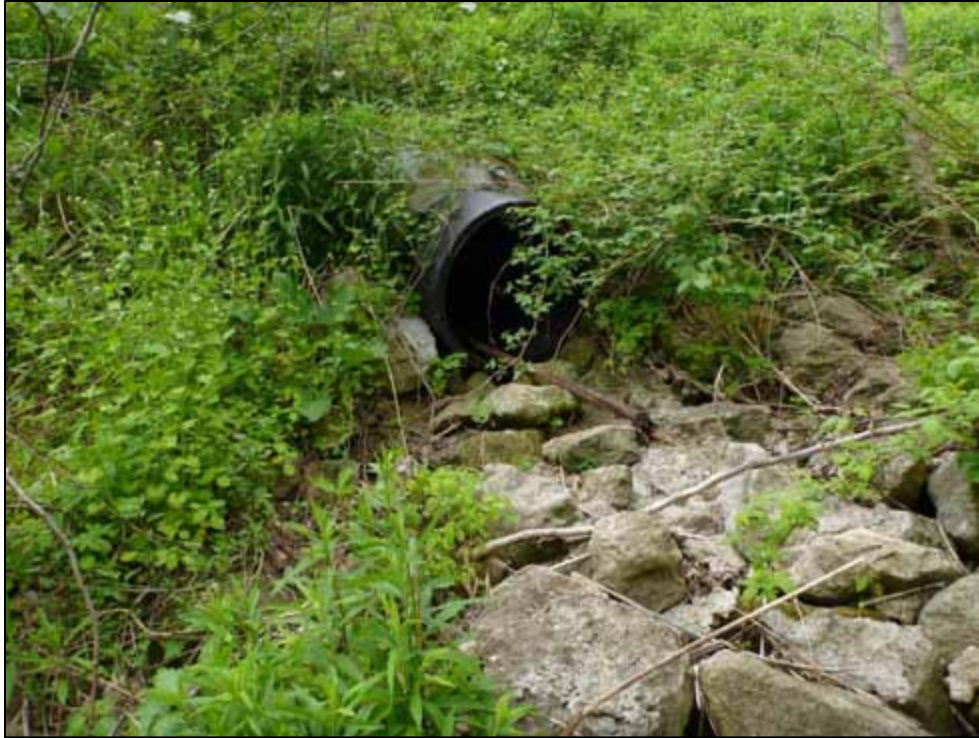
Photo 61: Culvert C15, downstream face (looking west)
