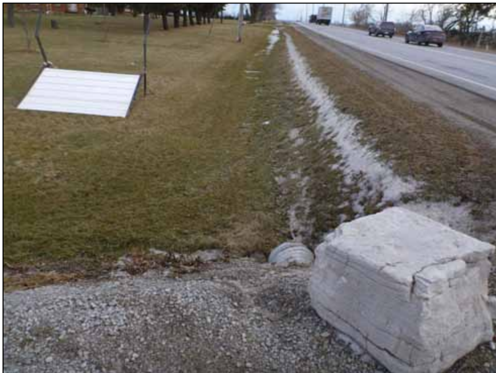
Photo 12: Culvert C3, upstream channel (looking east)
