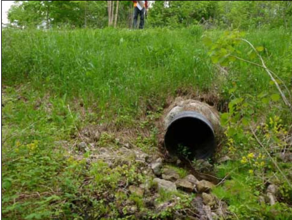
Photo 63: Culvert C15, upstream face (looking east)
