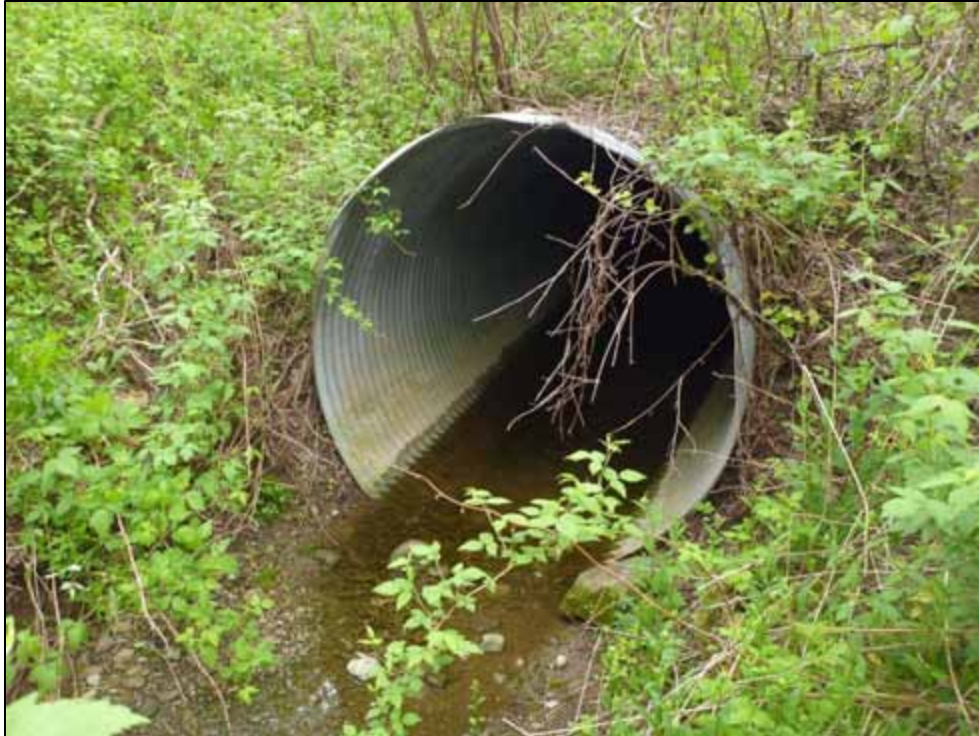
Photo 69: Culvert C16, downstream face (looking west)
