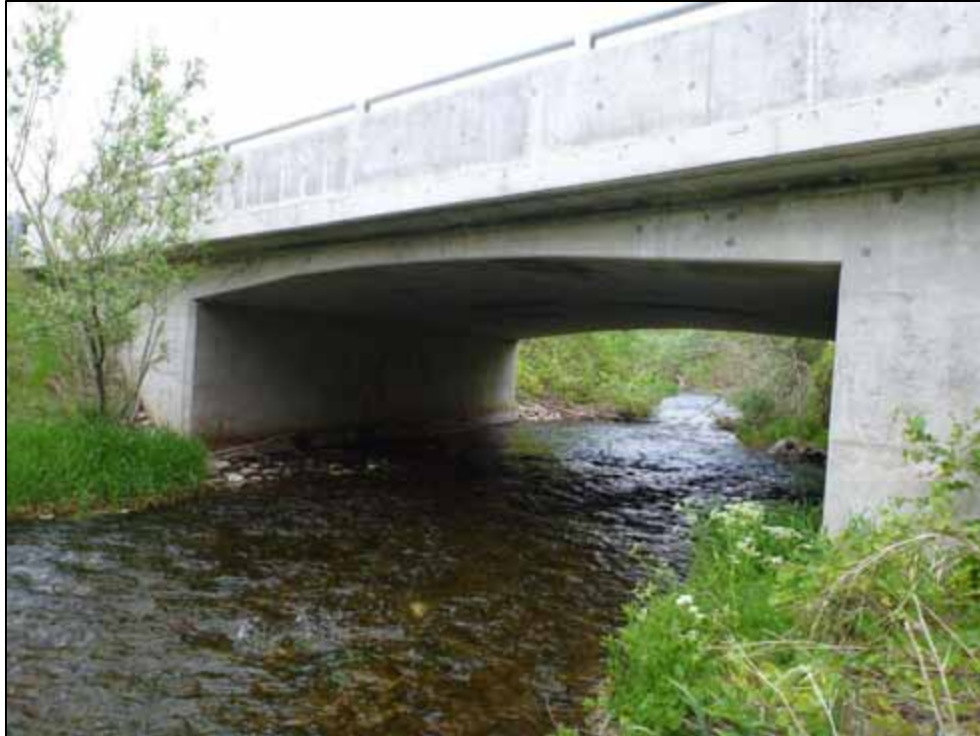
Photo 51: Bridge B1, upstream face (looking east)
