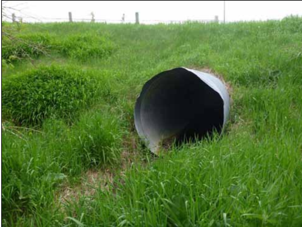
Photo 73: Culvert C18, downstream face (looking west)
