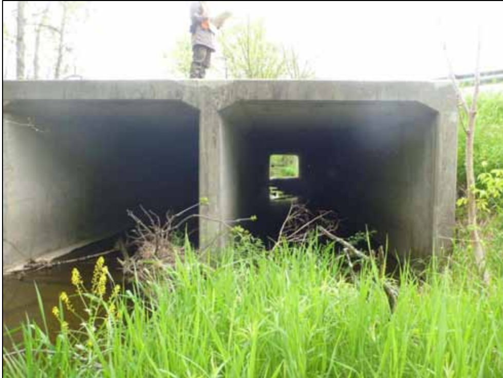
Photo 7: Culvert C2, upstream face (looking south)
