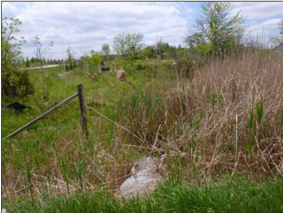
Photo 60: Culvert C14, upstream channel (looking west)
