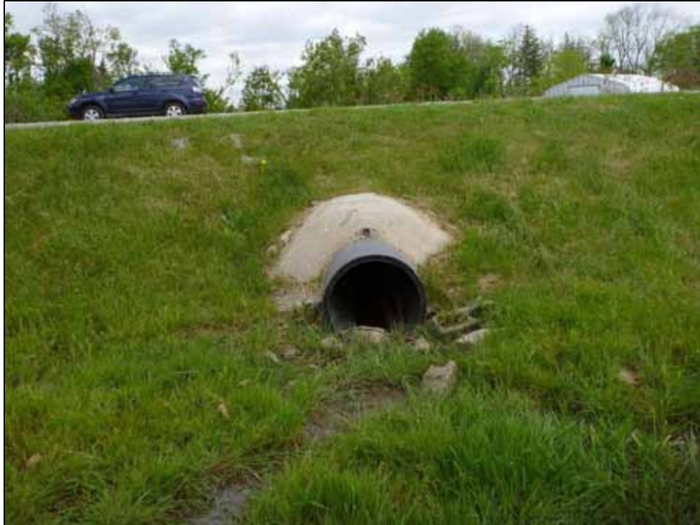
Photo 55: Culvert C13, upstream face (looking east)
