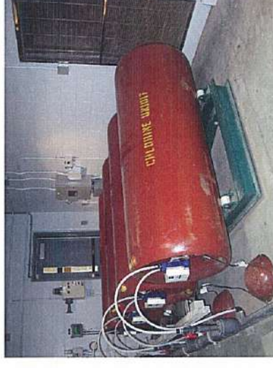
Chlorinators - Gas Cylinders
