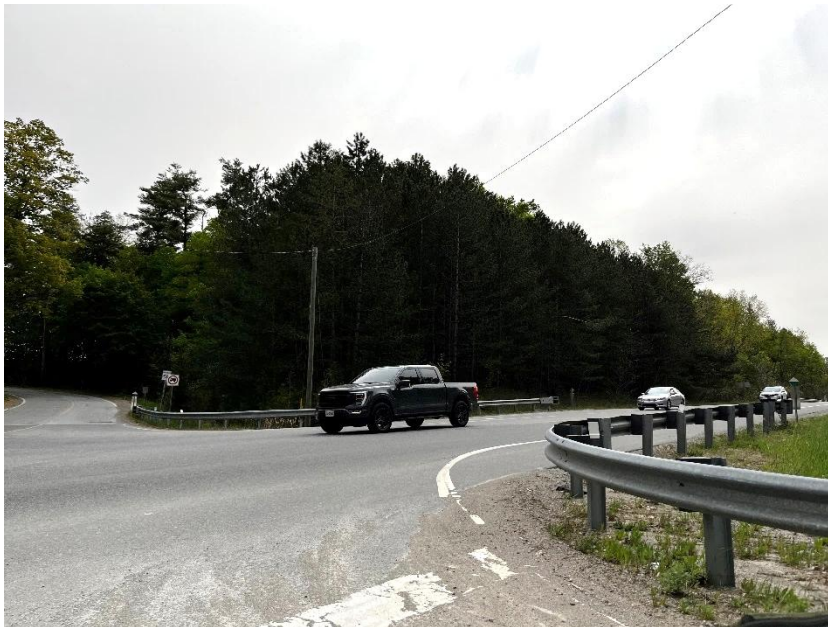
Plate 1: R.R. 25, looking east from the south side of 10 Side Road (A.S.I., 2023).
