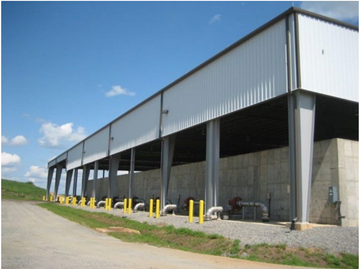
Figure 8-3. Example of Covered Aerated Static Pile System with Extended Aeration Stations
