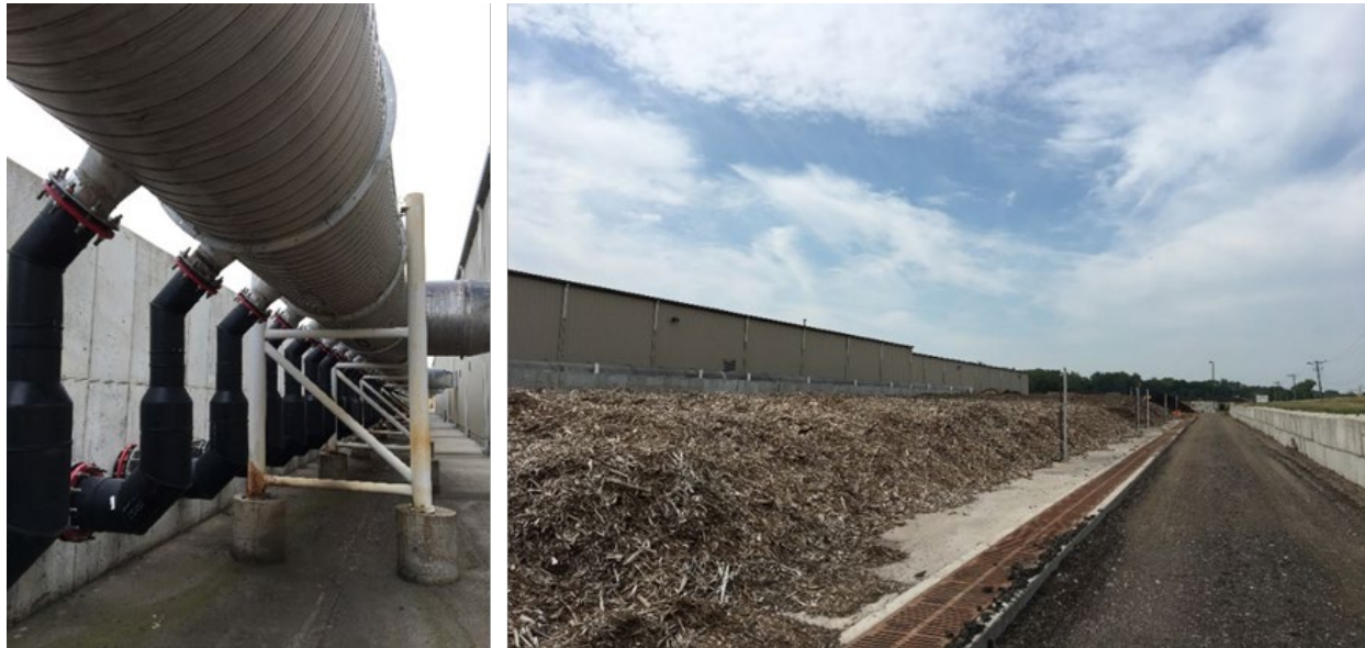
Figure 8-6. Example of Odour Control Collection Duct (left) and Biofilters (right)
