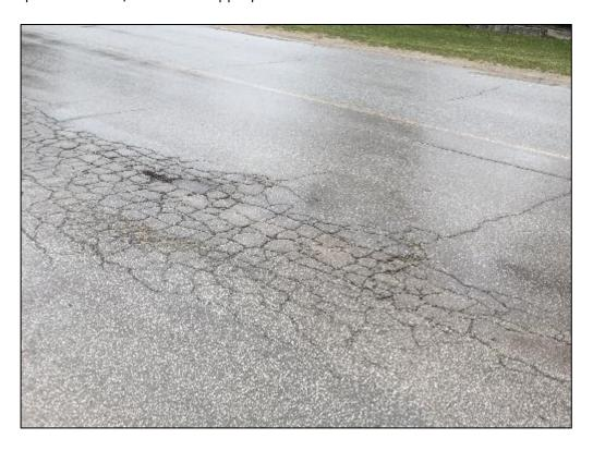
Figure 3: Example of poor pavement conditions on No 2 Side Road (TNS, 2021).
