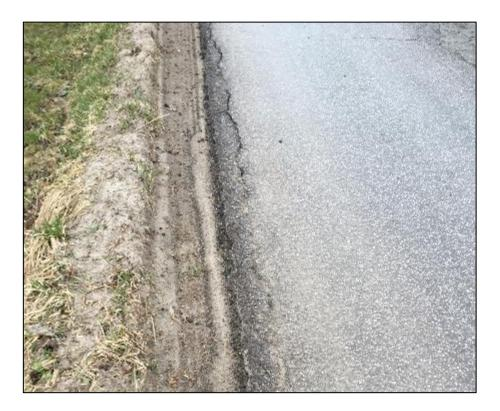
Figure 4: Example of pavement edge drop-off conditions on No 2 Side Road (TNS, 2021).
