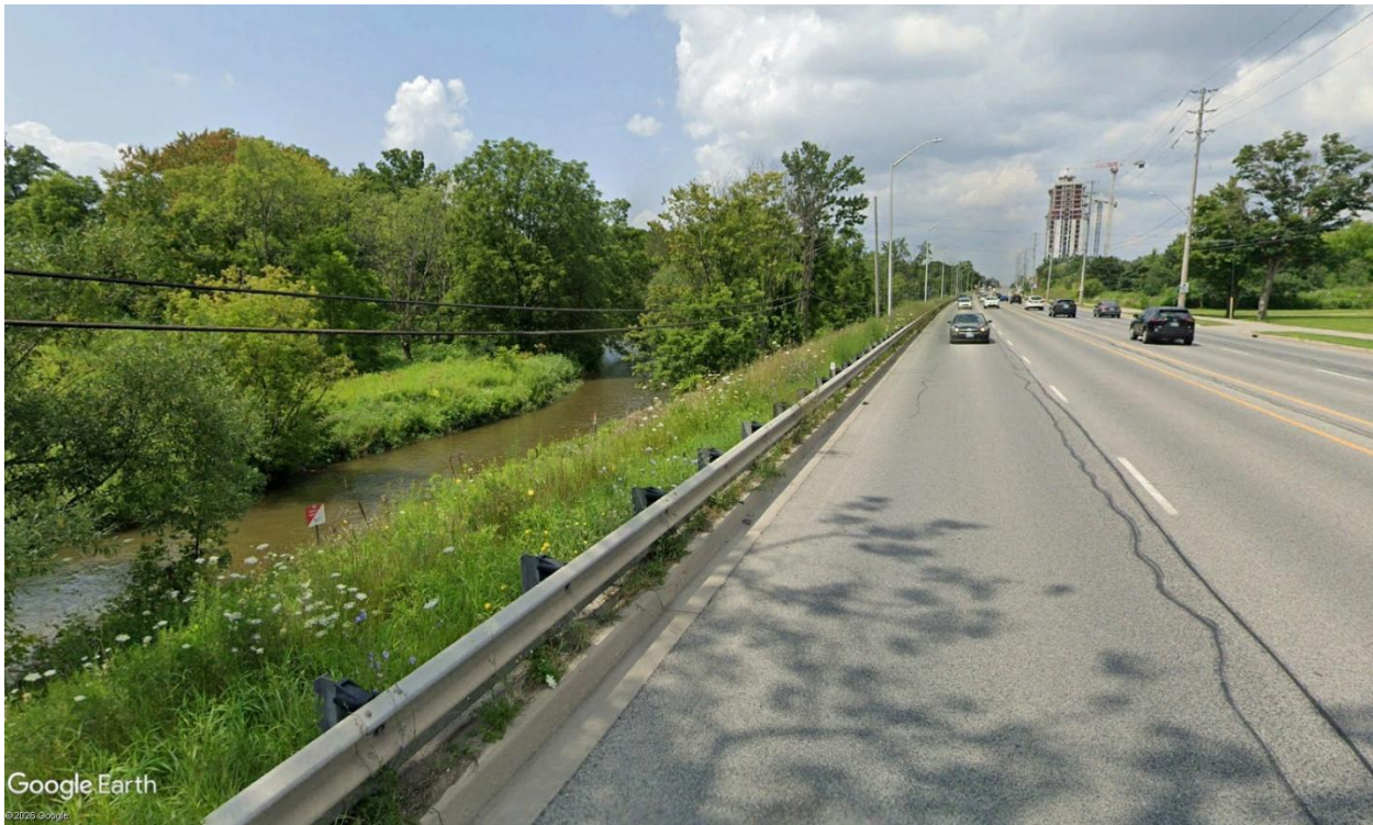
Figure 5-7: Regional Road 25 Near Sixteen Mile Creek (Looking North)
