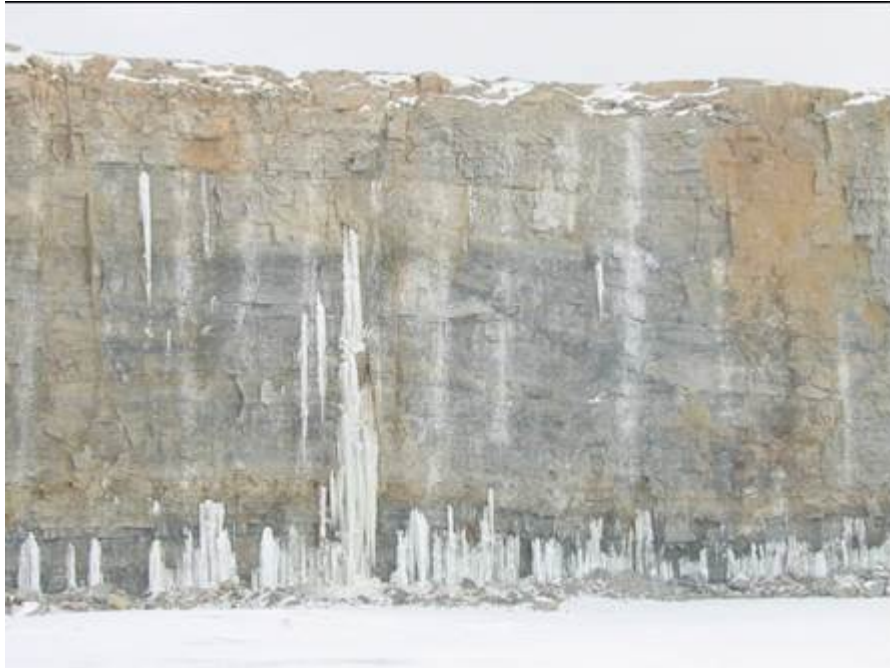
Figure 2. Multiple ice deposits near the base of the quarry wall and spare ice higher in the wall below the processing plant. The location is shown in Figure 1.
