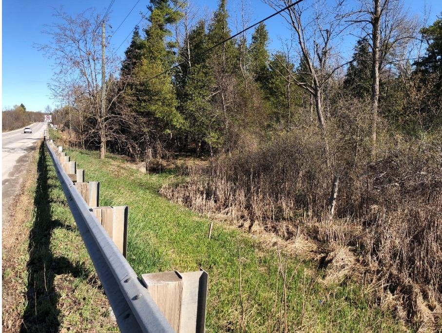
Image 15: Tributary channelized under the road, lands beyond disturbed road right-of-way require test pit survey.
