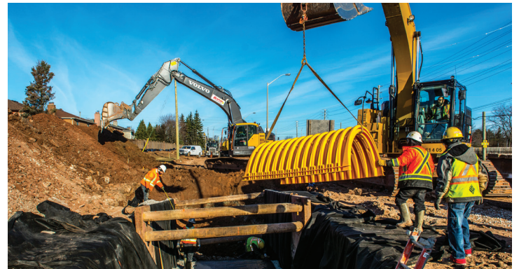
Image 1: Infiltration trenches, which help collect stormwater runoff, are installed south of Upper Middle Road.
