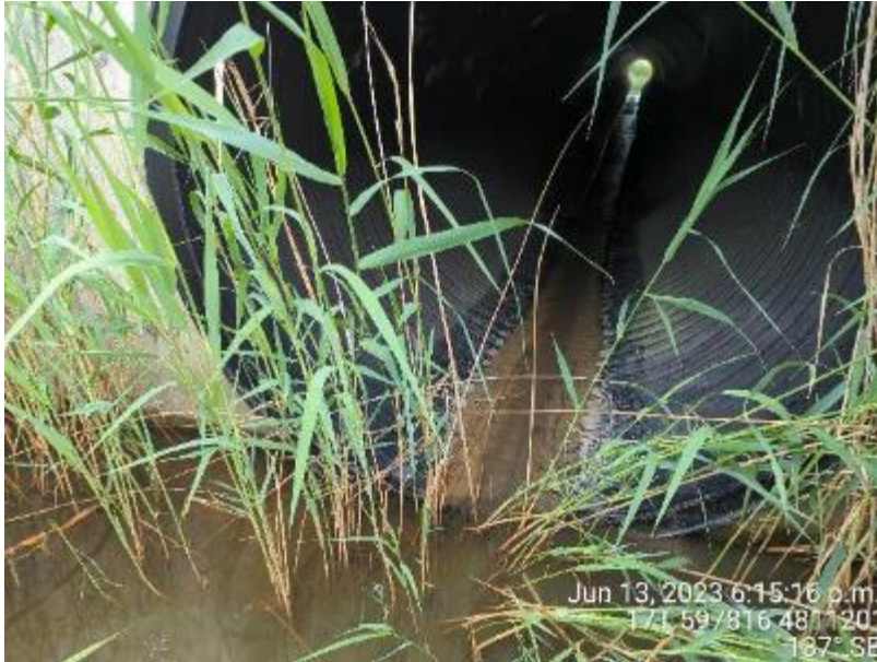
Figure 55: Looking downstream from the upstream end of the culvert (June 13, 2023)
