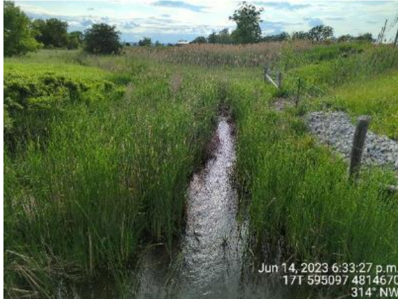
Figure 42: Looking upstream from the culvert at Regional Road 25 (June 14, 2023)
