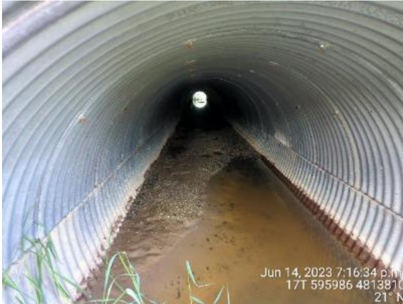
Figure 48: Looking downstream through the culvert (June 14, 2023)
