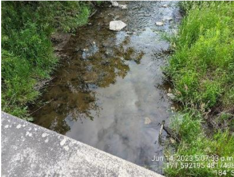
Figure 30: Looking downstream at the downstream end of the box culvert (June 14, 2023)
