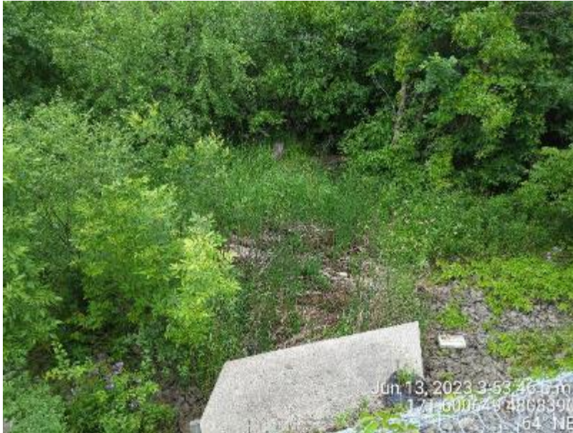
Figure 57: Looking downstream from Regional Road 25 (June 13, 2023)
