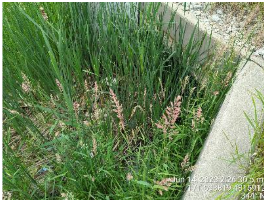
Figure 36: Looking at the downstream end of the culvert (June 14, 2023)
