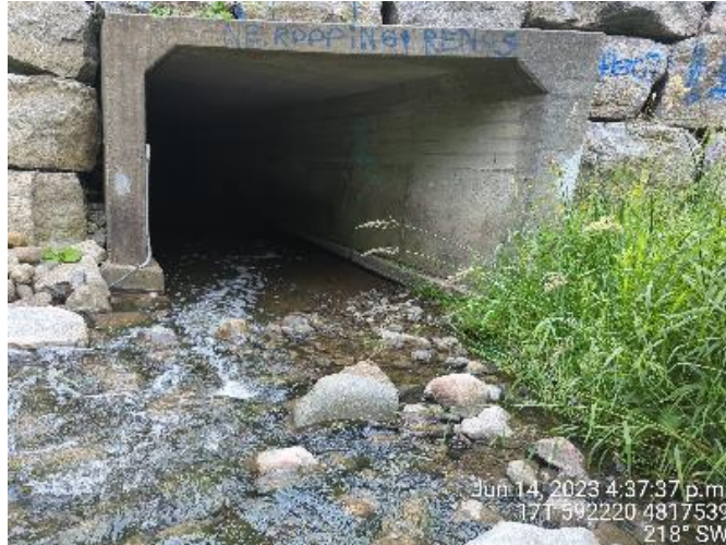
Figure 32: Looking upstream in the box culvert (June 14, 2023)
