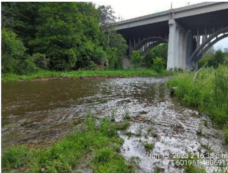
Figure 61: Looking upstream at Bronte Creek near Regional Road 25 (June 13, 2023)
