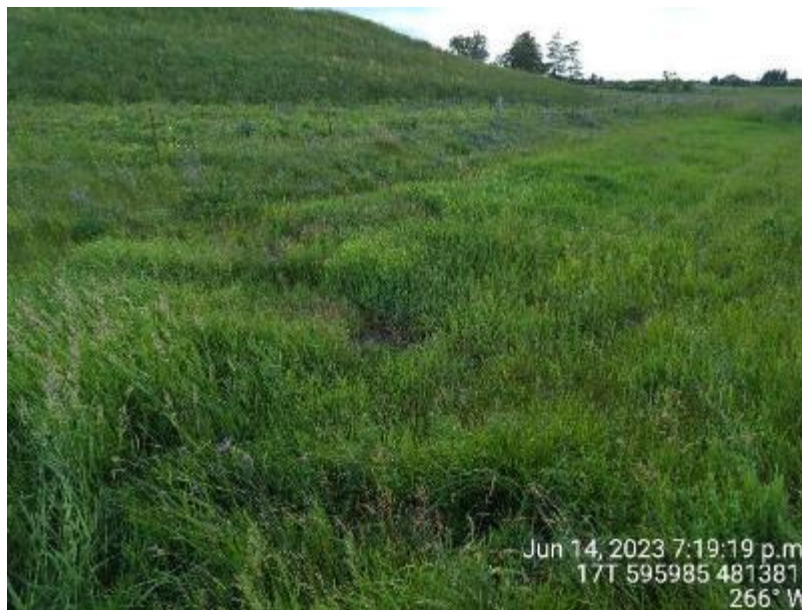
Figure 47: Looking upstream from the culvert at Regional Road 25 (June 14, 2023)
