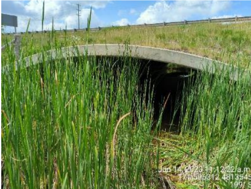
Figure 49: Looking upstream from the downstream end of the culvert (June 14, 2023)
