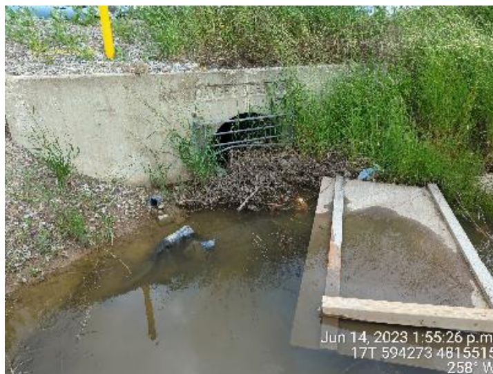
Figure 38: Looking at the upstream end of the culvert (June 14, 2023)
