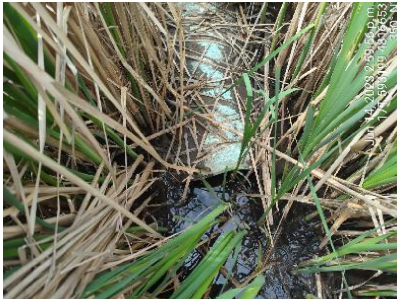
Figure 34: Looking at the upstream culvert (June 14, 2023)
