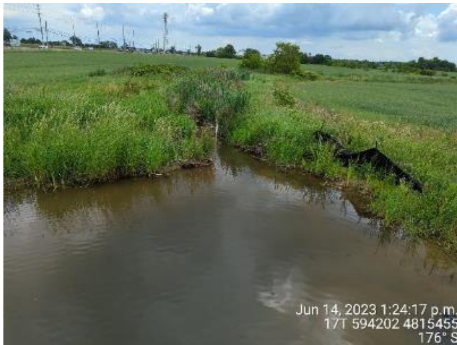
Figure 39: Looking downstream from the bridge at Britannia Road (June 14, 2023)
