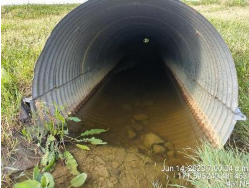
Figure 43: Looking downstream through the culvert at Regional Road 25 (June 14, 2023)
