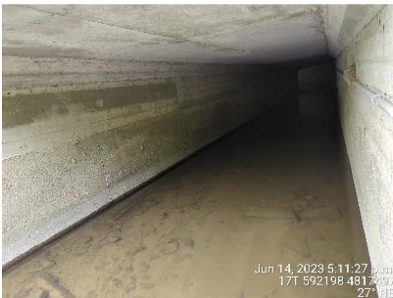
Figure 31: Looking upstream in the box culvert (June 14, 2023)
