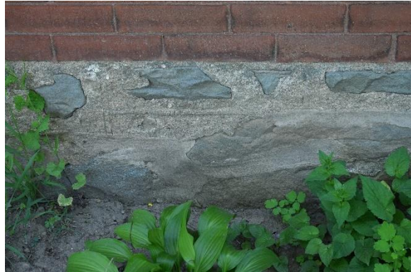
Photo 17 Representative photo of stone foundation
