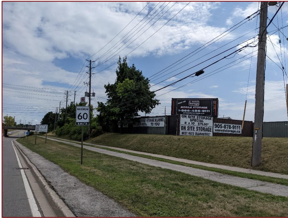
Image 4: Regional Road 25 South of QEW - Grading
