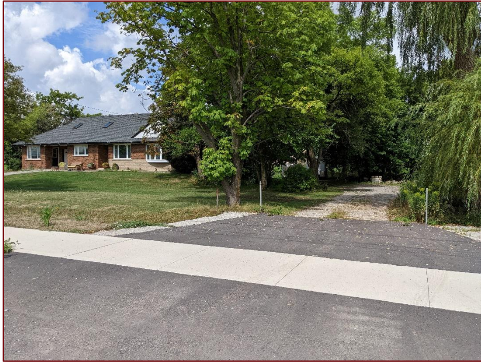
Image 54: Regional Road 25 at Ethridge Avenue – Sidewalk and New Intersection Construction
