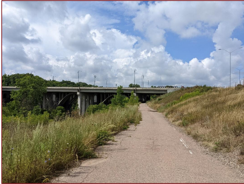
Image 6: West of Regional Road 25 at QEW Overpass – Grading Adjacent to Bronte Creek
