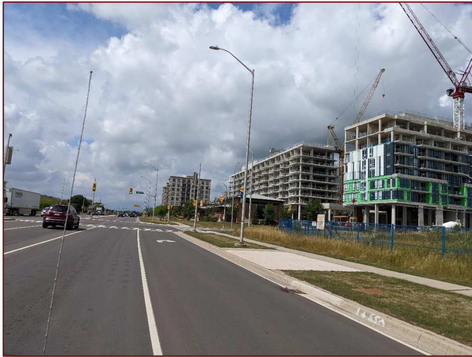
Image 24: West of Regional Road 25 South of Dundas Street West – Sidewalk and Grading
