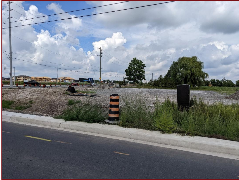
Image 52: Regional Road 25 North of Britannia Road – Graded for Creek Rehabilitation
